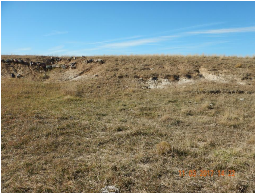
Photo 5. Photo taken from the western well pad location, facing West. Appears stormwater run-on onto the location is causing gully erosion along the western cut slope which is causing degradation to the location. Operator needs to repair gully erosion and install sufficient BMPs.
