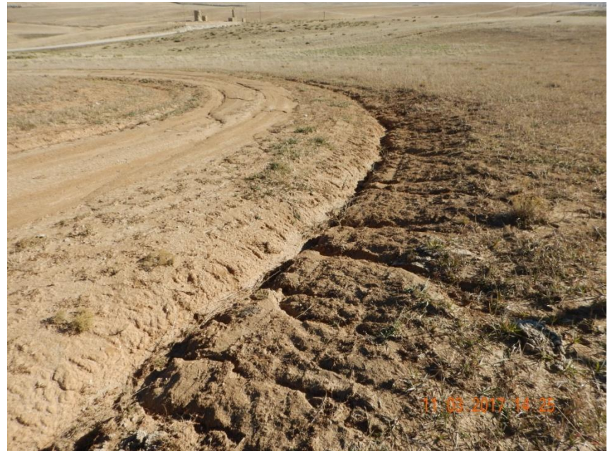
Photo 6. Photo taken from a portion of the access road, facing East. Rill erosion forming into gully erosion is evident along the access road. Operator needs to repair erosion and install sufficient BMPs.
