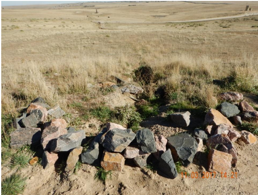
Photo 3. Photo taken from the northeast well pad, facing East. Rip-rap has been installed but does not appear to be a sufficient BMP as active gully erosion is evident. Operator needs to repair gully erosion and install sufficient BMPs.
