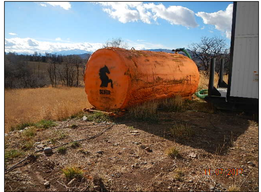
Photo 4. Sewer tank on edge of location. No down gradient controls.
