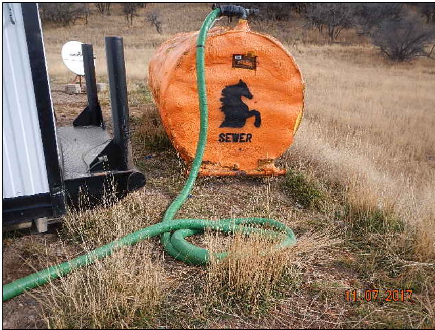
Photo 3. Sewer tank on edge of location. No down gradient controls.
