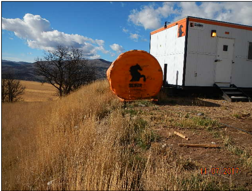
Photo 1. Sewer tank on edge of location. No down gradient controls.
