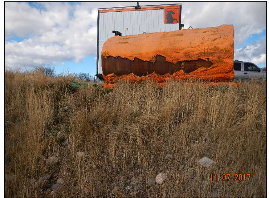
Photo 2. Sewer tank on edge of location. No down gradient controls.
