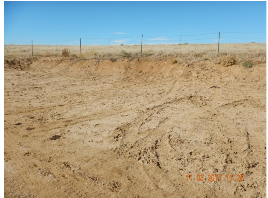
Photo 4. Photo taken November 3, 2017 from the previous photo location, facing Southwest. Does not appear the Operator has made repairs to the rill erosion along the cut slope. Does not appear the Operator has installed a BMP to prevent erosion and stabilize the production area.
