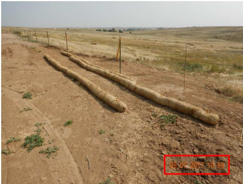
Photo 1. Photo taken September 7, 2017 from the eastern location where there was a previous gully erosion event, facing Northeast. Appears to Operator has repaired the erosion. Operator has installed wattle BMPs but BMP has not been properly installed and is not a sufficient BMP.
