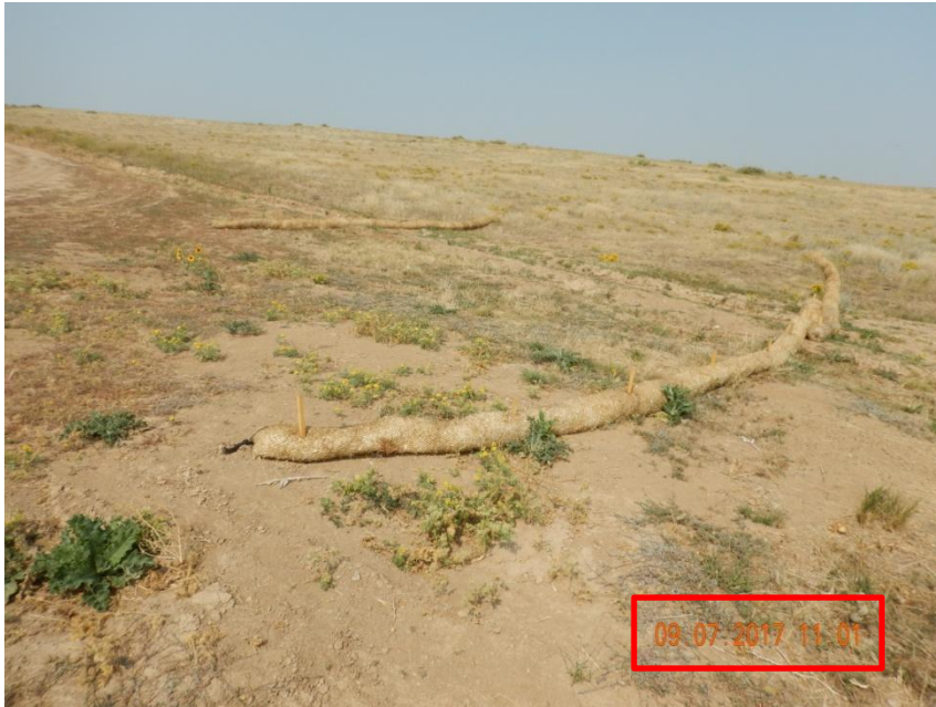
Photo 5. Photo taken September 7, 2017 from the second discharge point off the main access road, facing North. Operator has installed wattle BMPs but BMP has not been properly installed and is not a sufficient BMP.
