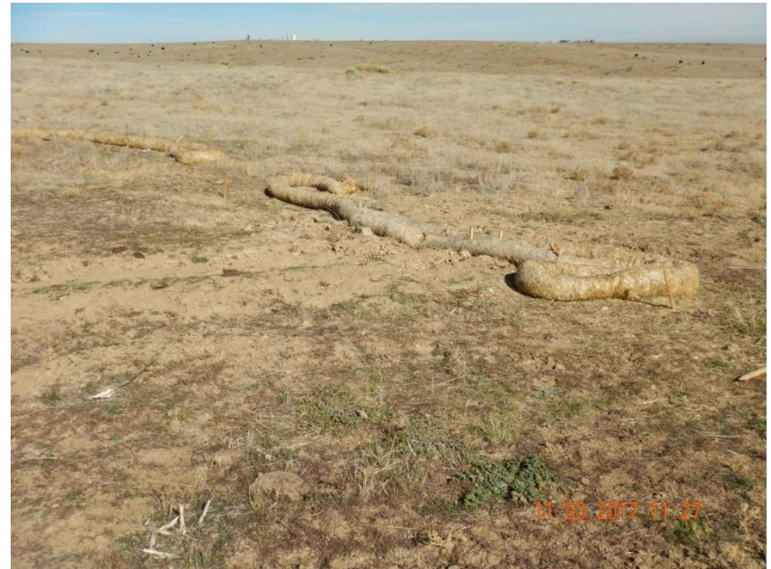
Photo 6. Photo taken November 3, 2017 from the previous photo location, facing North. Operator has not performed any further work to install sufficient BMPs. The wattle BMP has been damaged due to cattle and is not in proper functioning condition.
