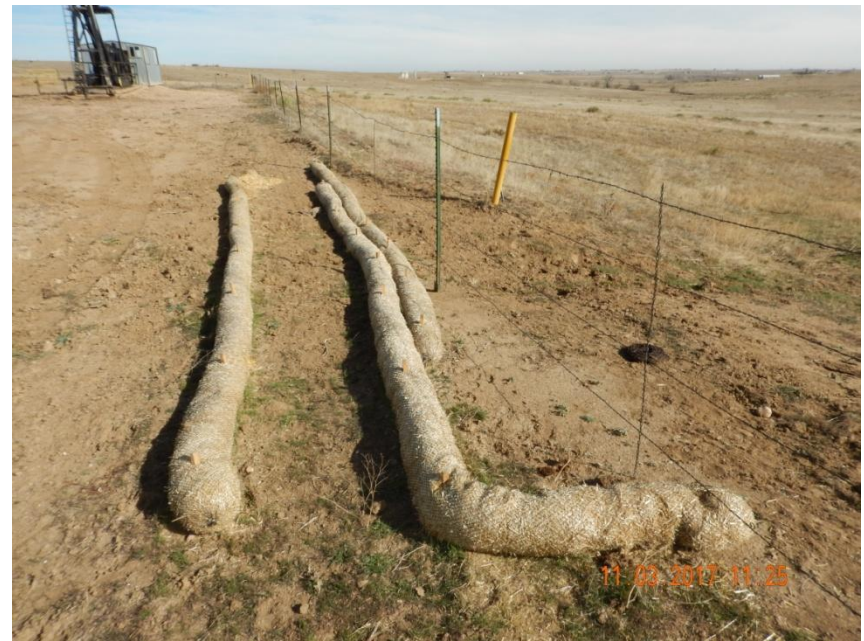
Photo 2. Photo taken November 3, 2017 from the previous photo location, facing North. Operator has not performed any further work to install sufficient BMPs. Portions of the wattle BMP have been damaged due to cattle.
