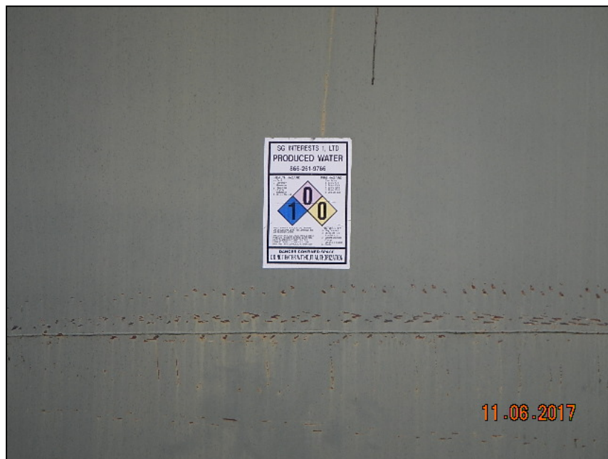
Photo 1. No capacity listed on tank. Update NFPA diamond for Produced Water or provide documentation for 0 fire hazard rating
