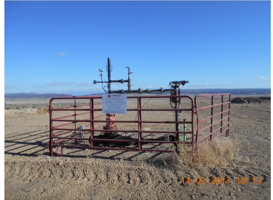
Wellhead with unused riser not locked out/tagged out/plugged.
