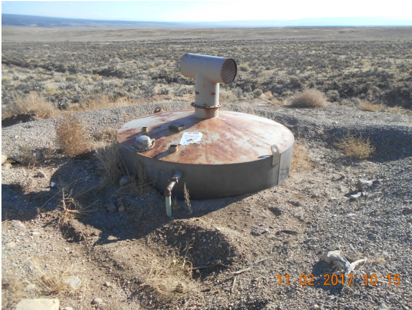
Tank with open pipe inlets.
