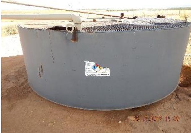
**Photo 5: Produced water tank with peeling NFPA label and no capacity label. Previous inspection.**
