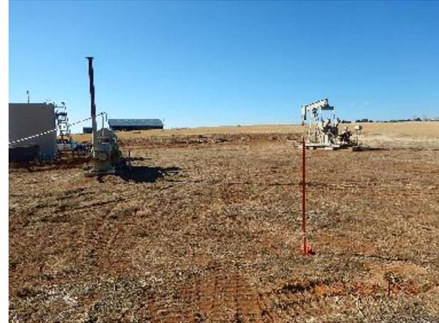
**Photo 12: Removed weeds and marked deadman. Follow-up inspection.**
