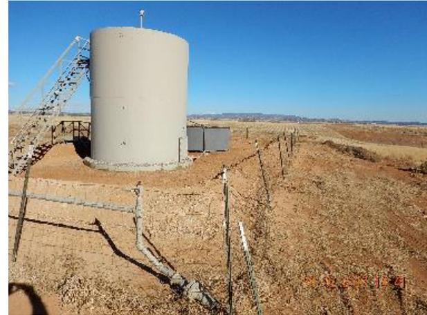
**Photo 14: Removed weeds and repaired berms. Follow-up inspection.**
