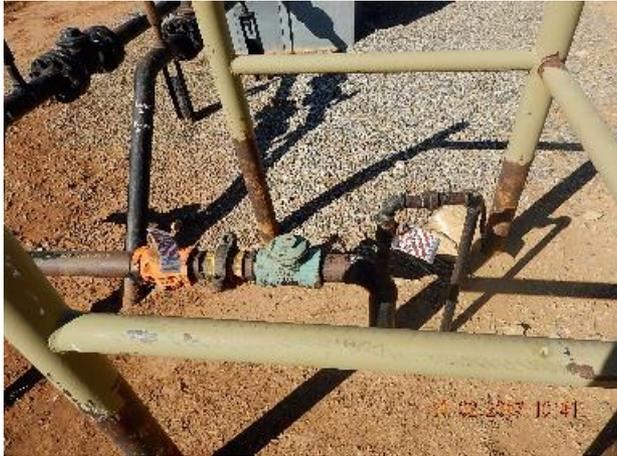
**Photo 7: Locked out tagged out lines at dog leg by gas meter run. Follow-up inspection.**
