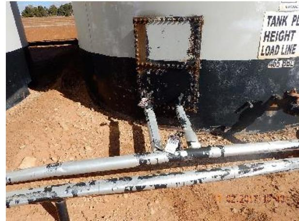
**Photo 8: Locked out and tagged out lines at production tank. Follow-up inspection.**
