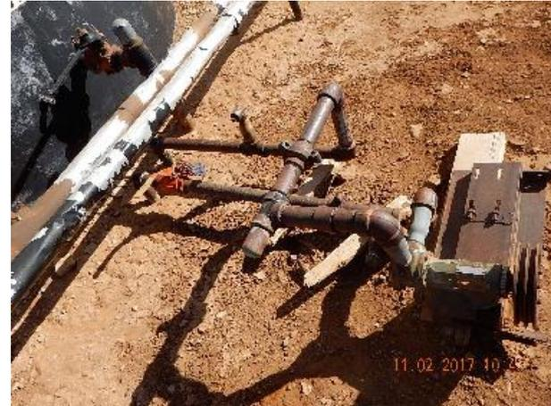
**Photo 4: Locked and tagged out lines at recirculating pump. Follow-up inspection.**
