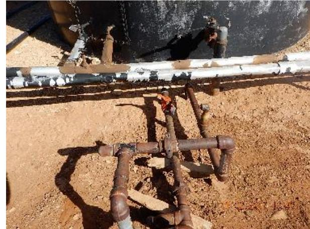
Photo 6: Locked out and tagged out recirculating lines at oil tank battery. Follow-up inspection.
