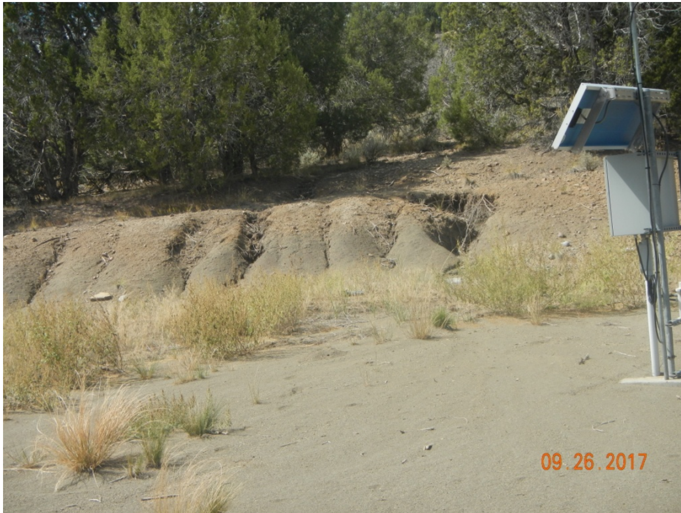
Photo 4. View of the eastern portion of the project area from the southeastern corner facing northward. Erosion is occurring within the western cut-slope. Stabilization is needed.
