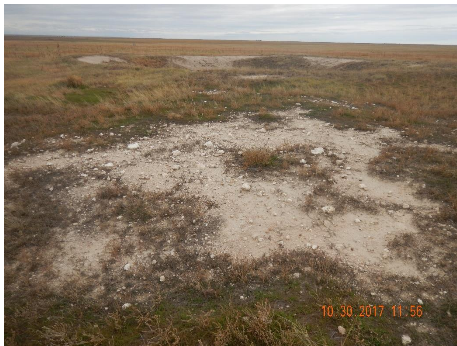
Photo 2: Photo taken from the southeast end of the well location, facing northwest. Photo shows well location remains predominantly unvegetated, and pit remains open. Unable to find evidence that reclamation activities have been conducted.
