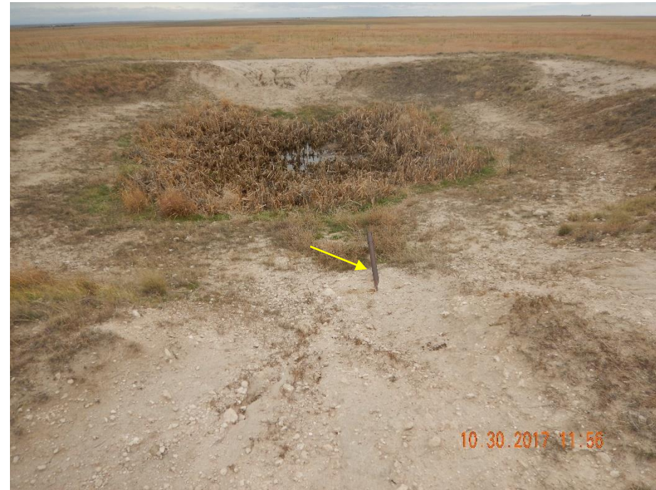
Photo 4: Photo taken from the east end of the pit location, facing west. Photo shows pit remains open and pipe remain.
