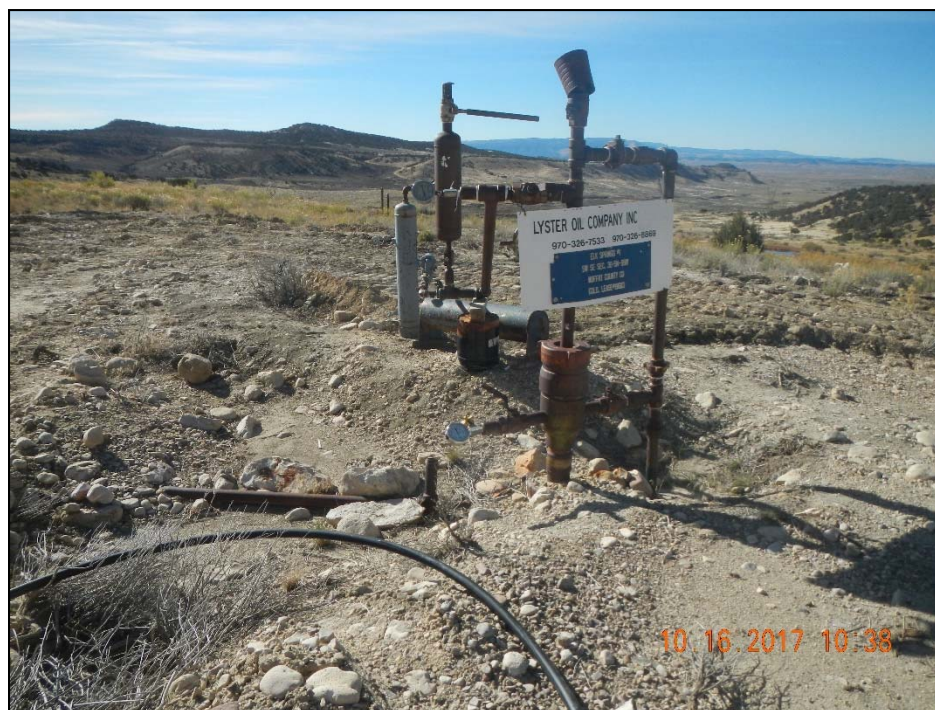
Photo 1. Overview of location facing southwest. 1" flowline at wellhead, 3 additional risers in background on left.
