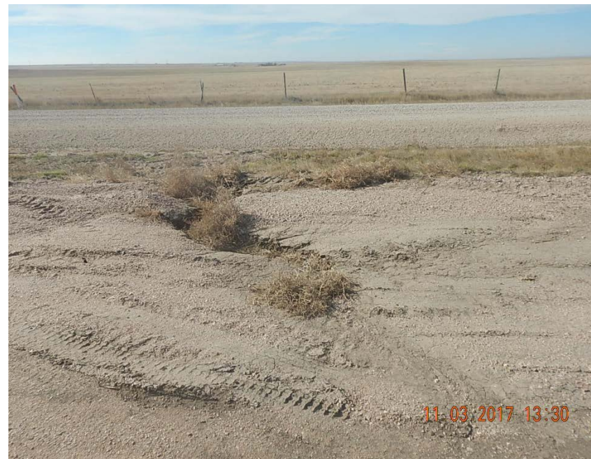
Photo 6: Stormwater erosion on W side of location
