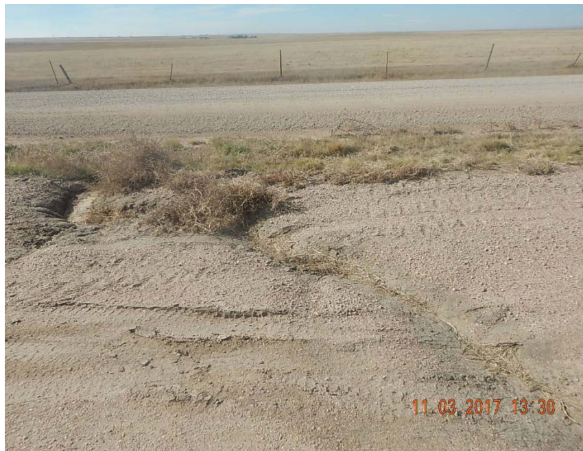
Stormwater erosion on W side of location
