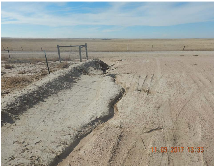
Photo 5: Stormwater erosion on SW corner of location
