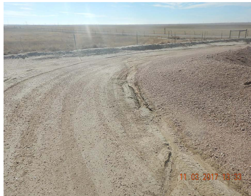
Photo 4: Stormwater on SE corner of battery berm
