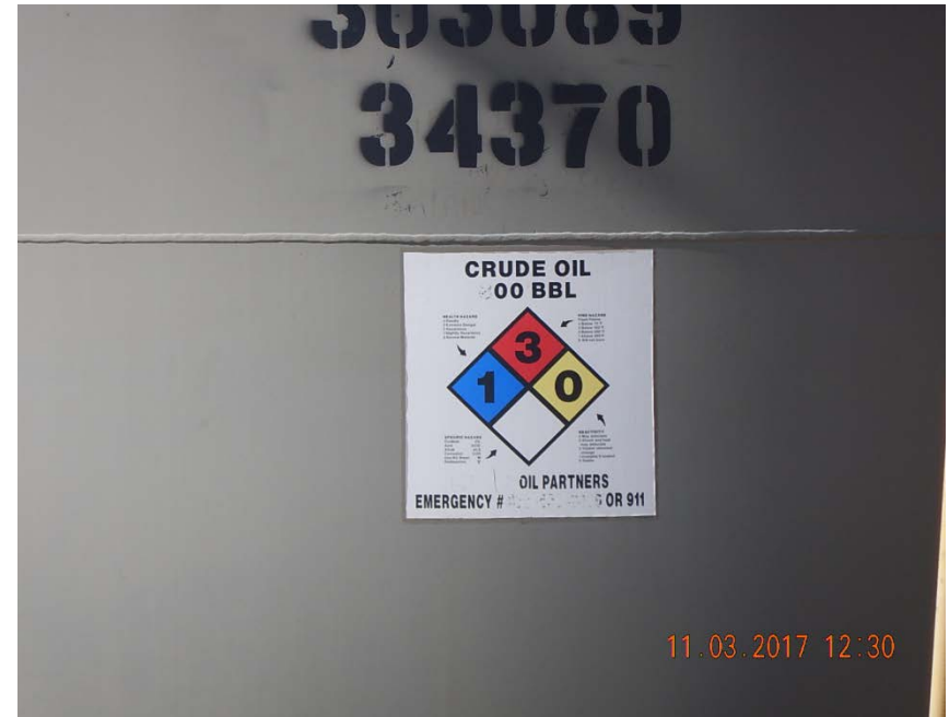
Photo 4: No capacity on crude oil decal
