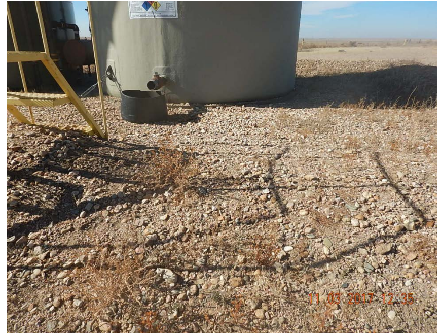
Photo 6: Berms eroded low, some weeds in battery
