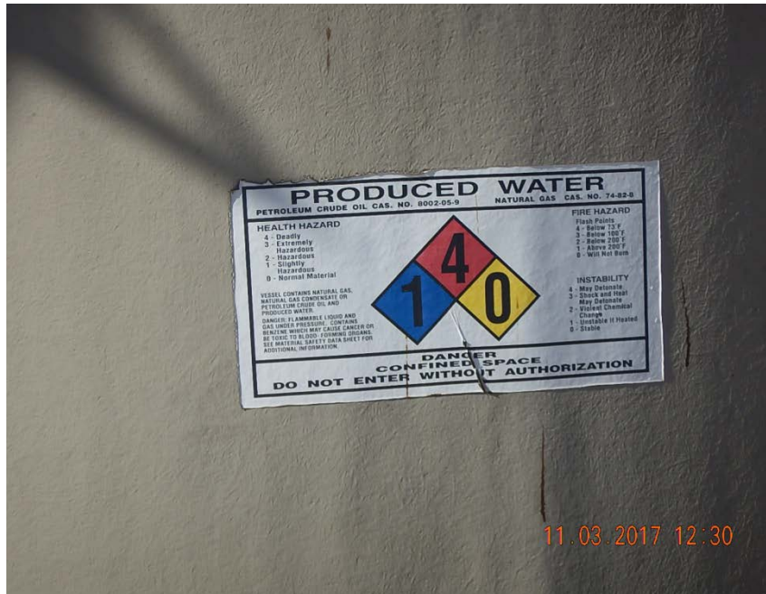
Photo 3: No capacity on produced water decal
