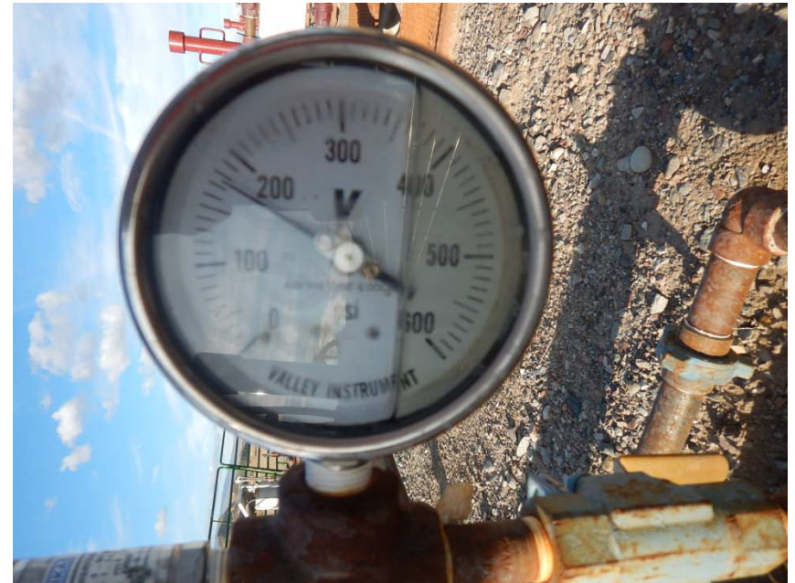
Gage on bradenhead manifold
