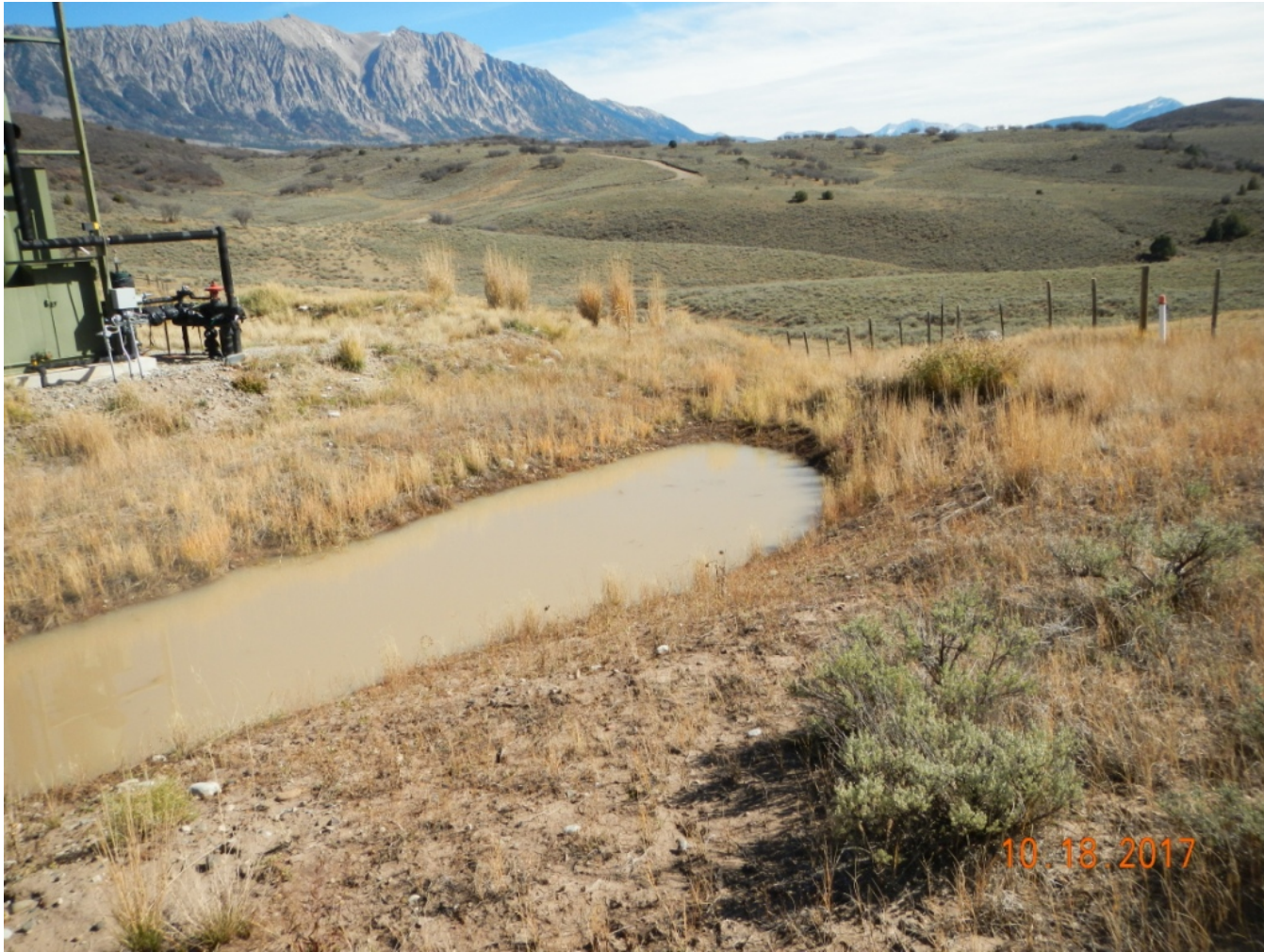
Photo 7. View of silt trap in good condition in the southern portion of the project area.
