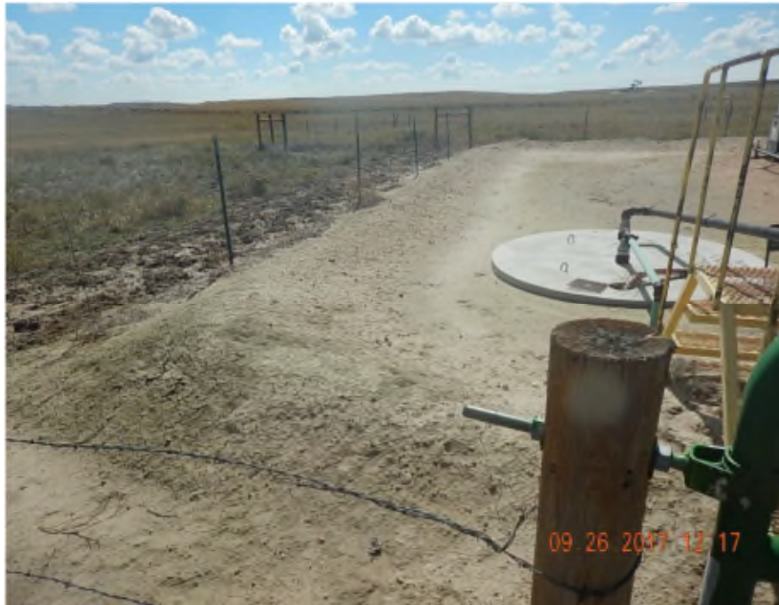
Photo 3: Low berms at tank battery
