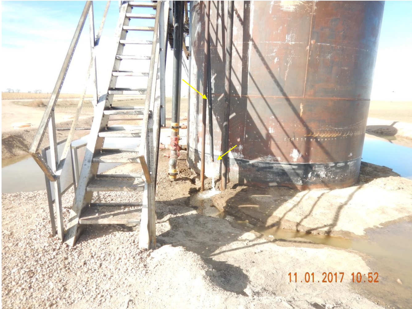
Photo 2: Photo taken from the east side of the produced water tank. Photo shows produced water is being discharged via the overflow-siphon line and into the containment berm.
