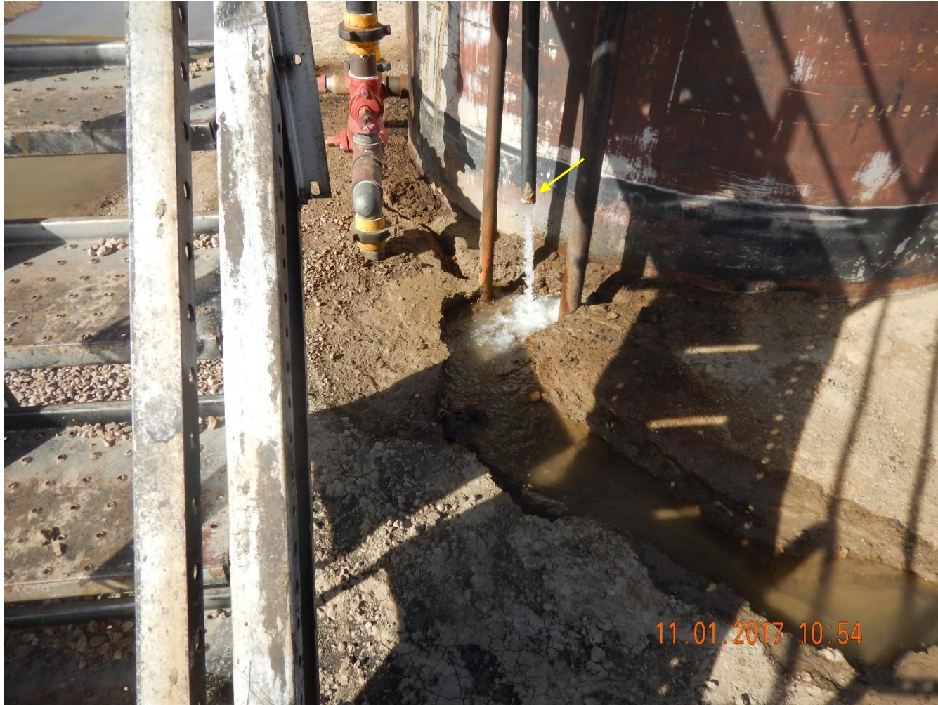
Photo 3: Photo taken from the east side of the produced water tank. Photo shows produced water is being discharged via the overflow-siphon line and into the containment berm.
