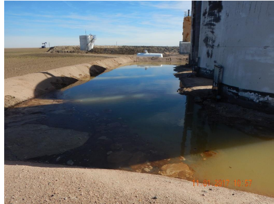
Photo 7: Photo taken from the west end of the battery. Photo shows produced water discharged into the containment berm. Photo also shows oil residue.
