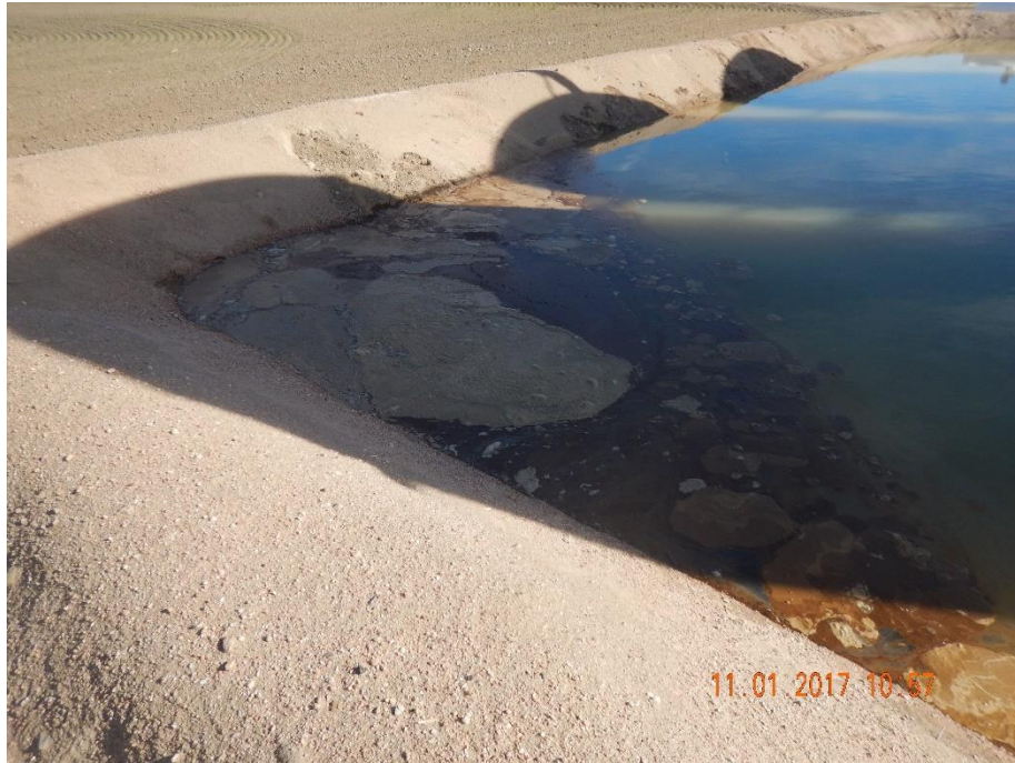
Photo 6: Photo taken from the west end of the battery. Photo shows produced water discharged into the containment berm. Photo also shows oil residue.
