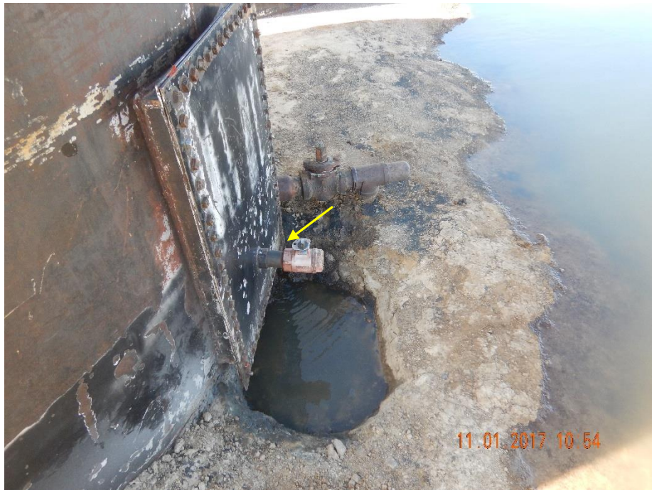
Photo 4: Photo taken from the north end of the produced water tank. Photo shows a leak occurring at the base of the manifold. This will require repair.
