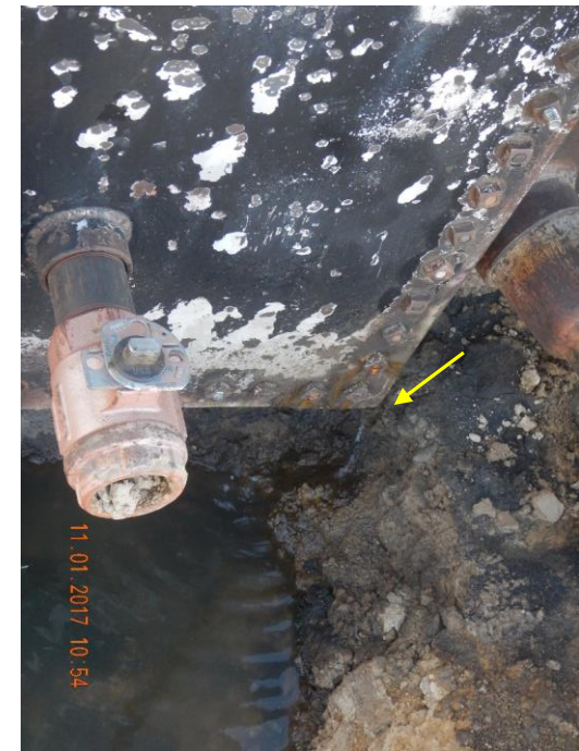
Photo 5: Photo taken from the north end of the produced water tank. Photo shows a leak occurring at the base of the manifold. This will require repair.
