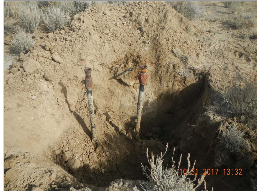
Photo 2. Excavation of flowlines.
