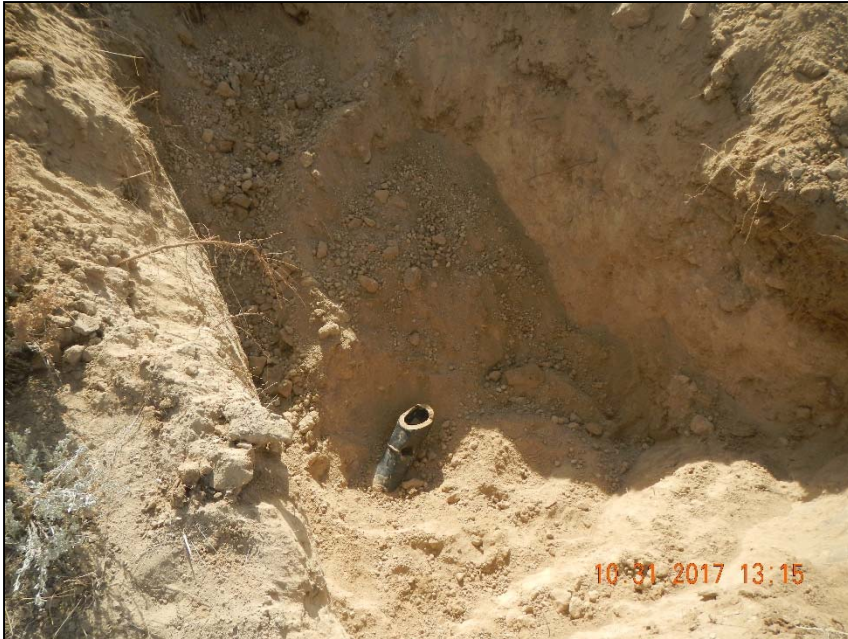
Photo 1. Excavation of flowlines.
