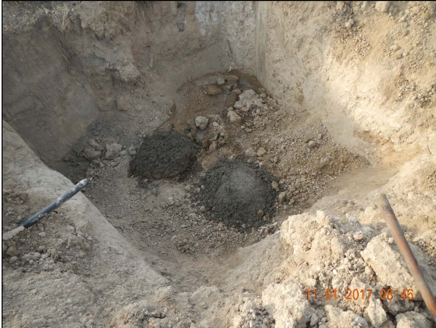
Photo 5. Surface of cement plugs.
