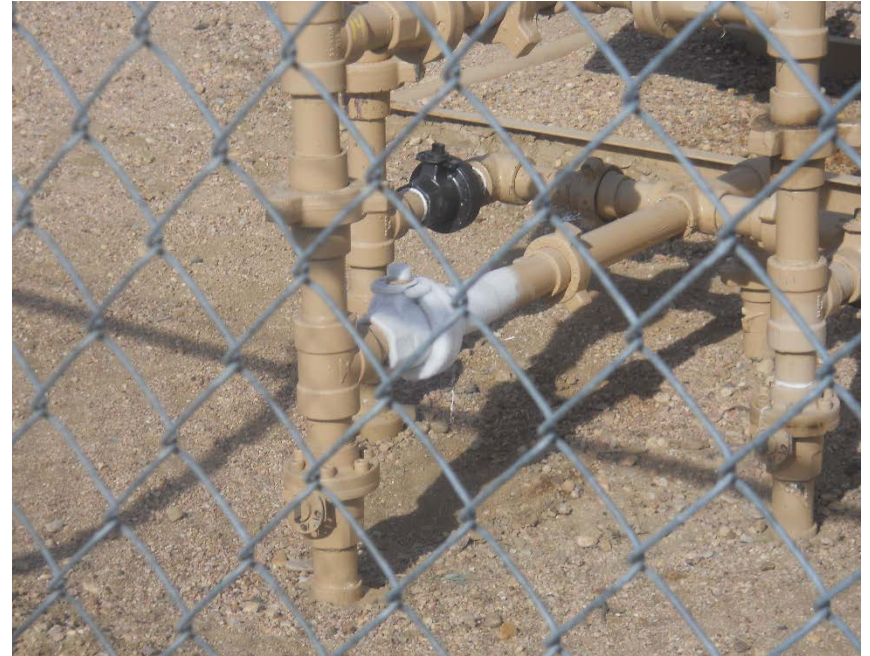
2" Balon bypass valve at separator header appears to be leaking by, frozen over
