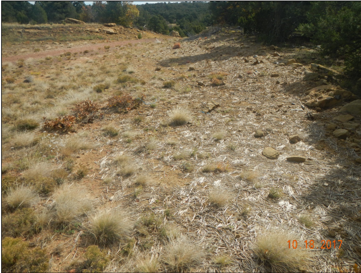
Photo 5. Facing east toward the south side of the location. Wood straw mulch has been applied to bare soil areas.
