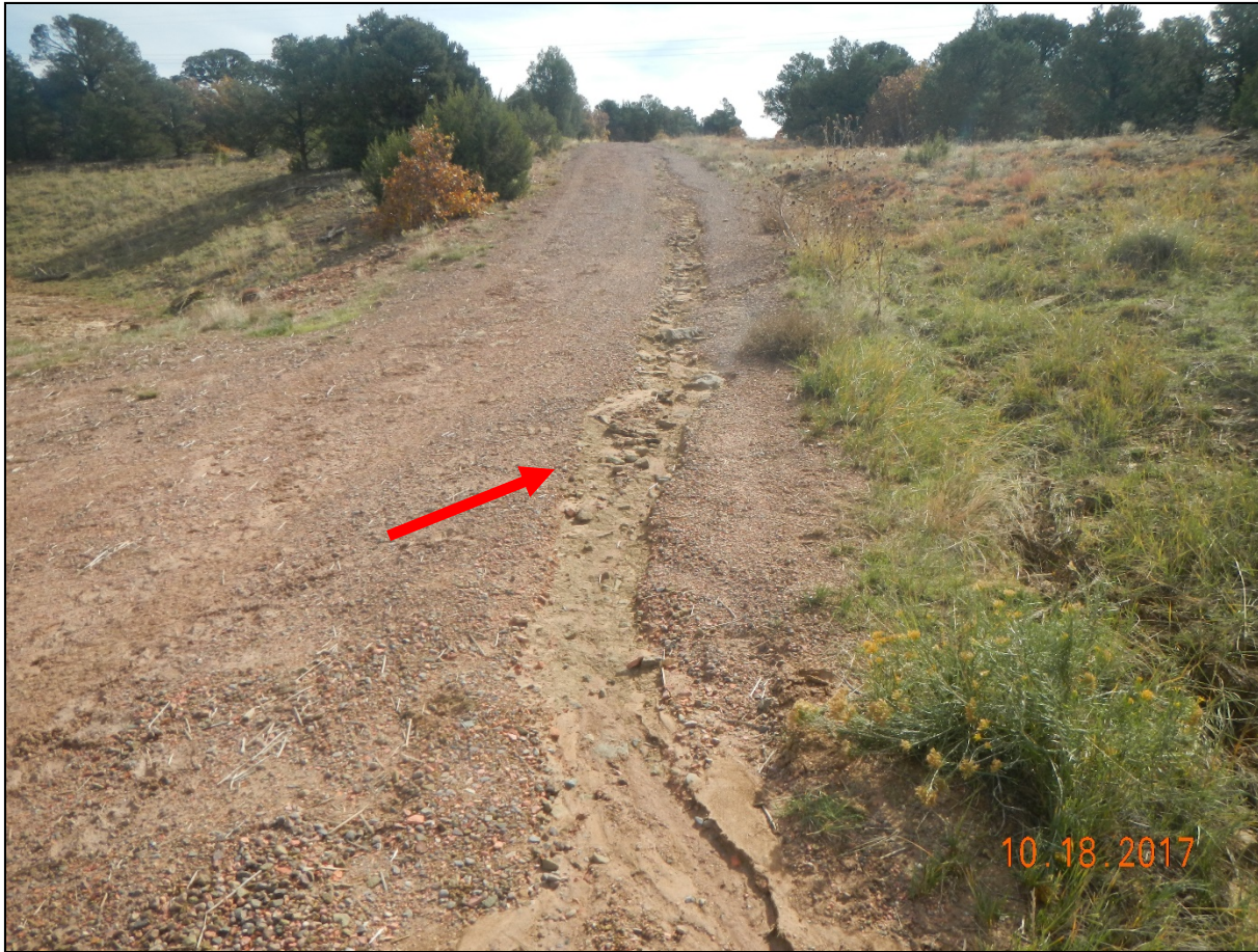
Photo 1. Facing southeast along the access road. There are signs of erosion occurring down the road.
