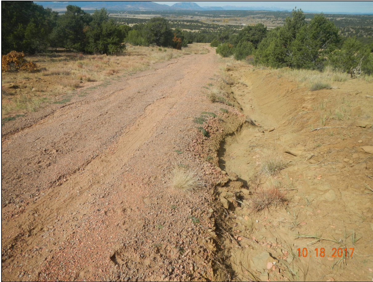
Photo 2. Facing back northwest along the access road. There is stormwater erosion occurring along the side of the road and no BMP's are installed.
