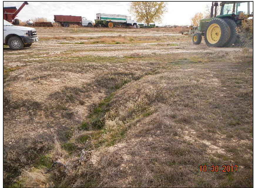
Photo 2. Erosion of location down gradient of wellhead. No stormwater controls in place.
