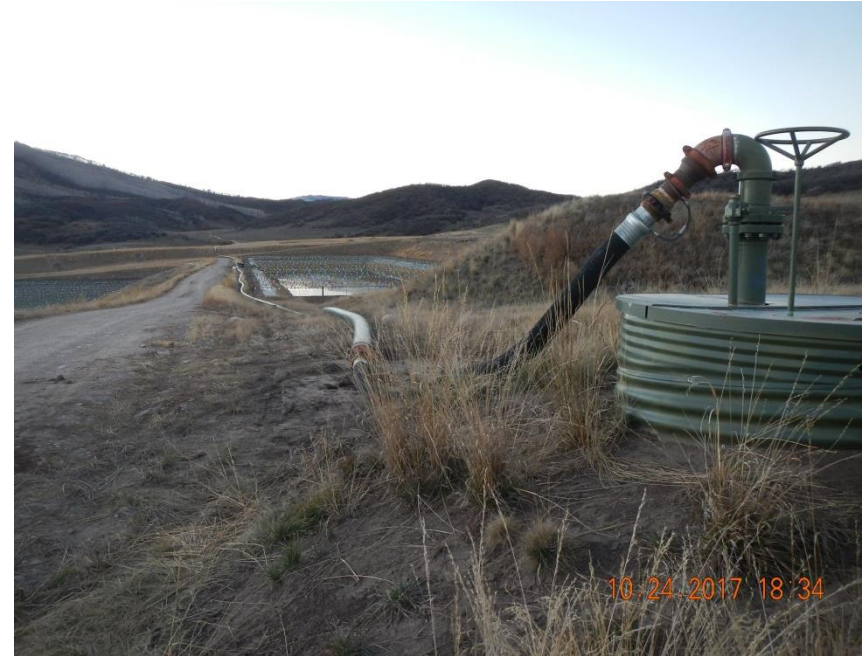
Pipe line valve can and water transfer line.
