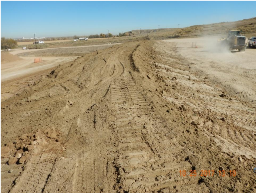
Photo 3. Photo taken from the north stockpile located on the middle tier, facing East. Material from the sediment basin is being spread onto the north stockpile and other stormwater erosion areas.
