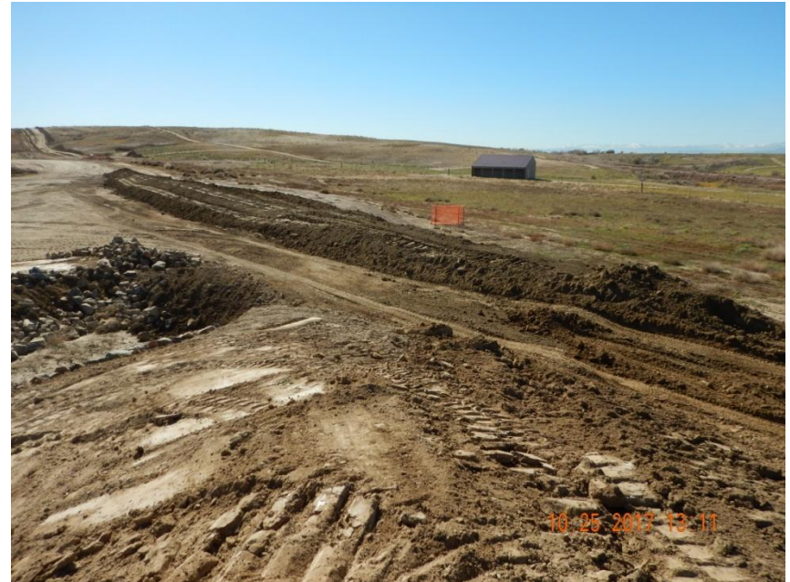
Photo 4. Photo taken from the north stockpile located on the middle tier, facing West. Stormwater construction work in process along the western location. Appears a berm is being constructed and the western access road has been removed.
