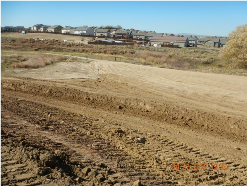
Photo 1. Photo taken from the north stockpile located on the middle tier, facing Northwest. Northwestern area appears to have been re-graded to direct stormwater flows east towards the sediment basin.
