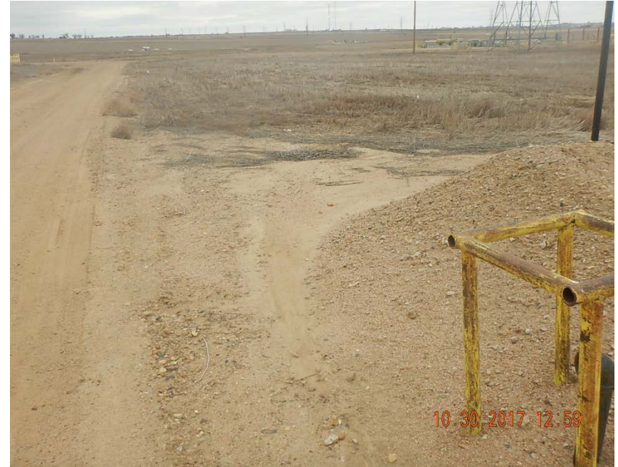
Photo 9: Stormwater erosion NW of battery
