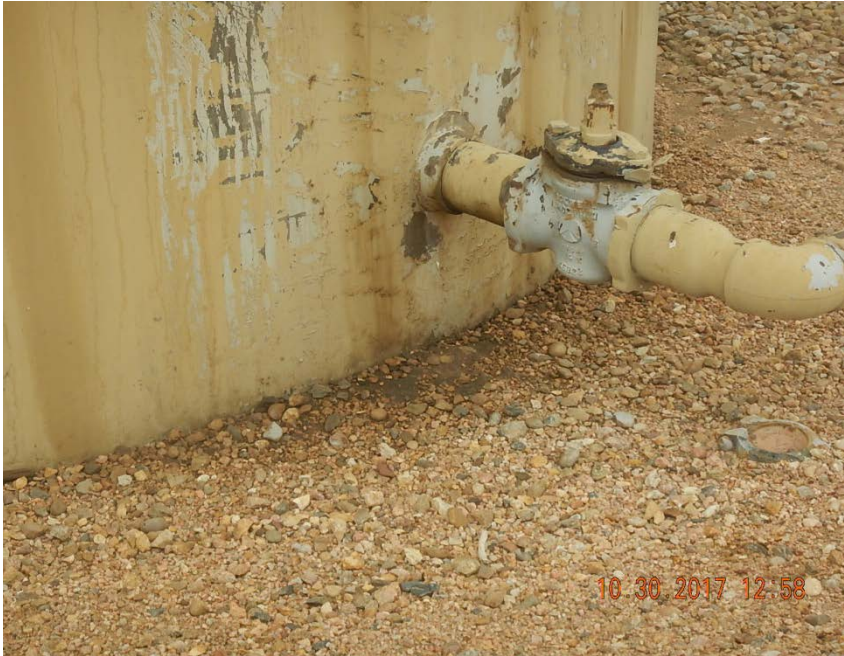
Photo 8: Stained soil at oil tank
