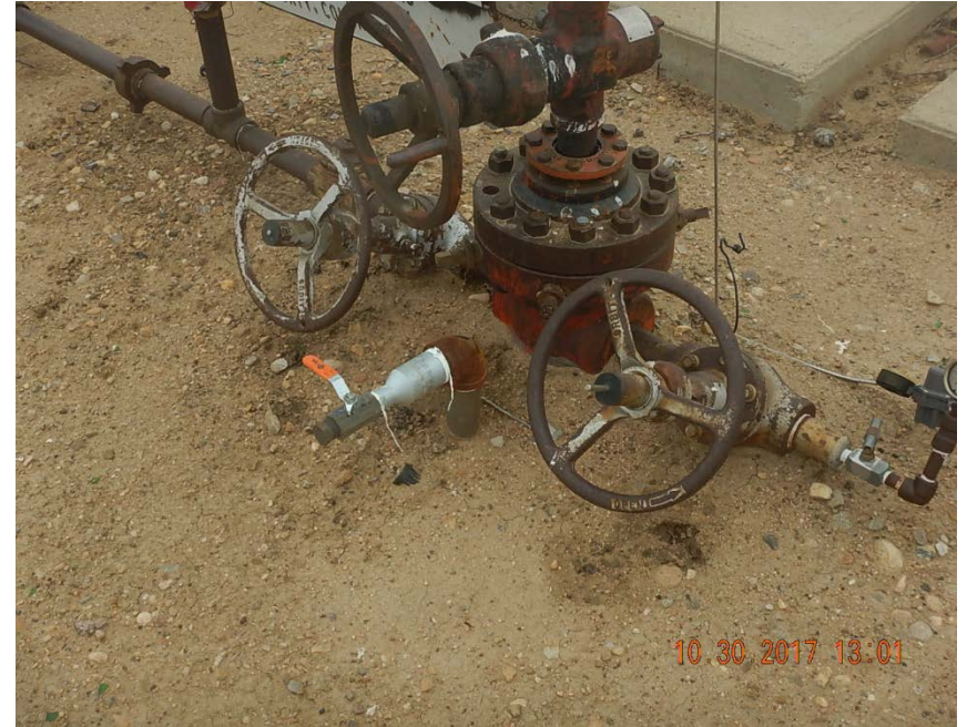
Photo 6: Bradenhead plumbed to surface.
