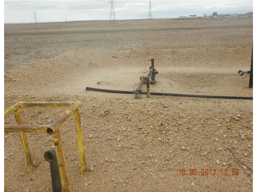
Photo 4: Produced water vault has no contents, capacities, safety labeling
