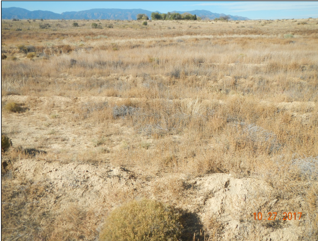
Photo 5. Facing west at the location. The location is not recontoured and there are rows of soil piled up on the surface.
