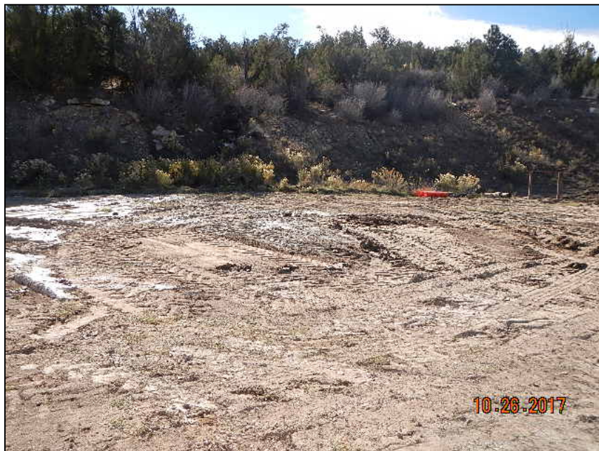
Photo 1. Wellhead has been cut off and buried after plugging.
