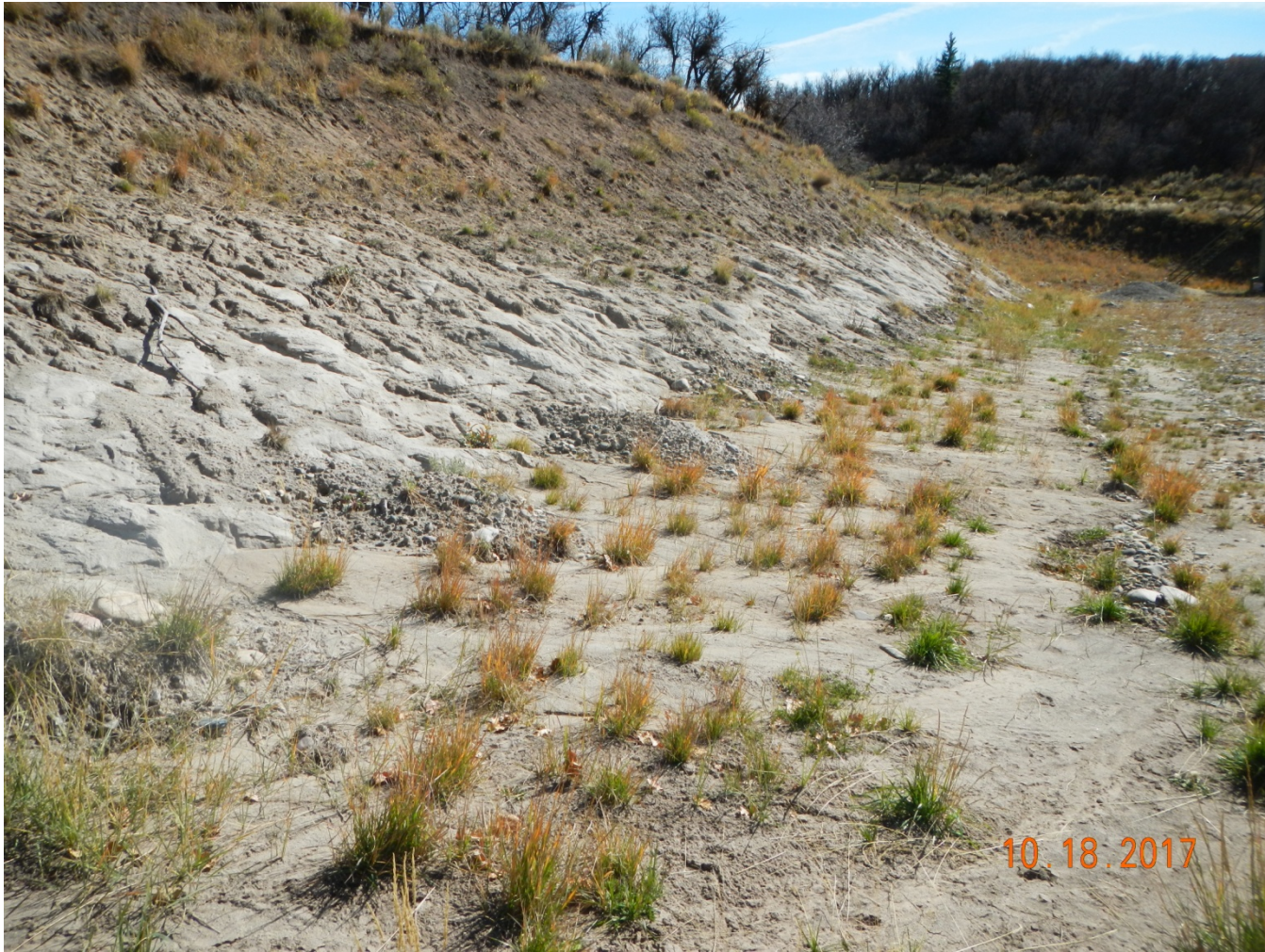
Photo 4. View of the eastern cut-slope from the northeastern corner facing southward. This slope is not stabilized as evidenced by the exposed roots at the top of the slope, erosional rilling within the slope, and sediment deposition at the toe of the slope.
