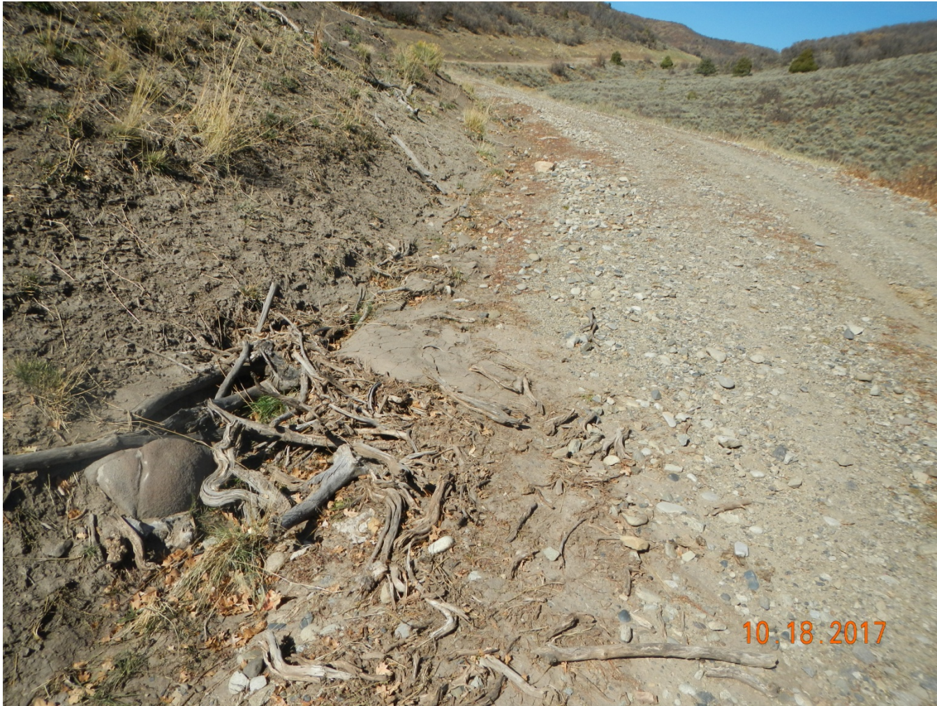
Photo 5. View of sediment deposition along the western edge of the access road, near the entrance to the access road facing northward.
