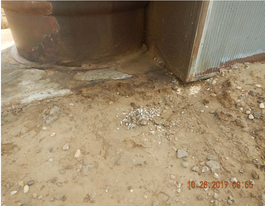
Photo 11: Stained soil at vessel
