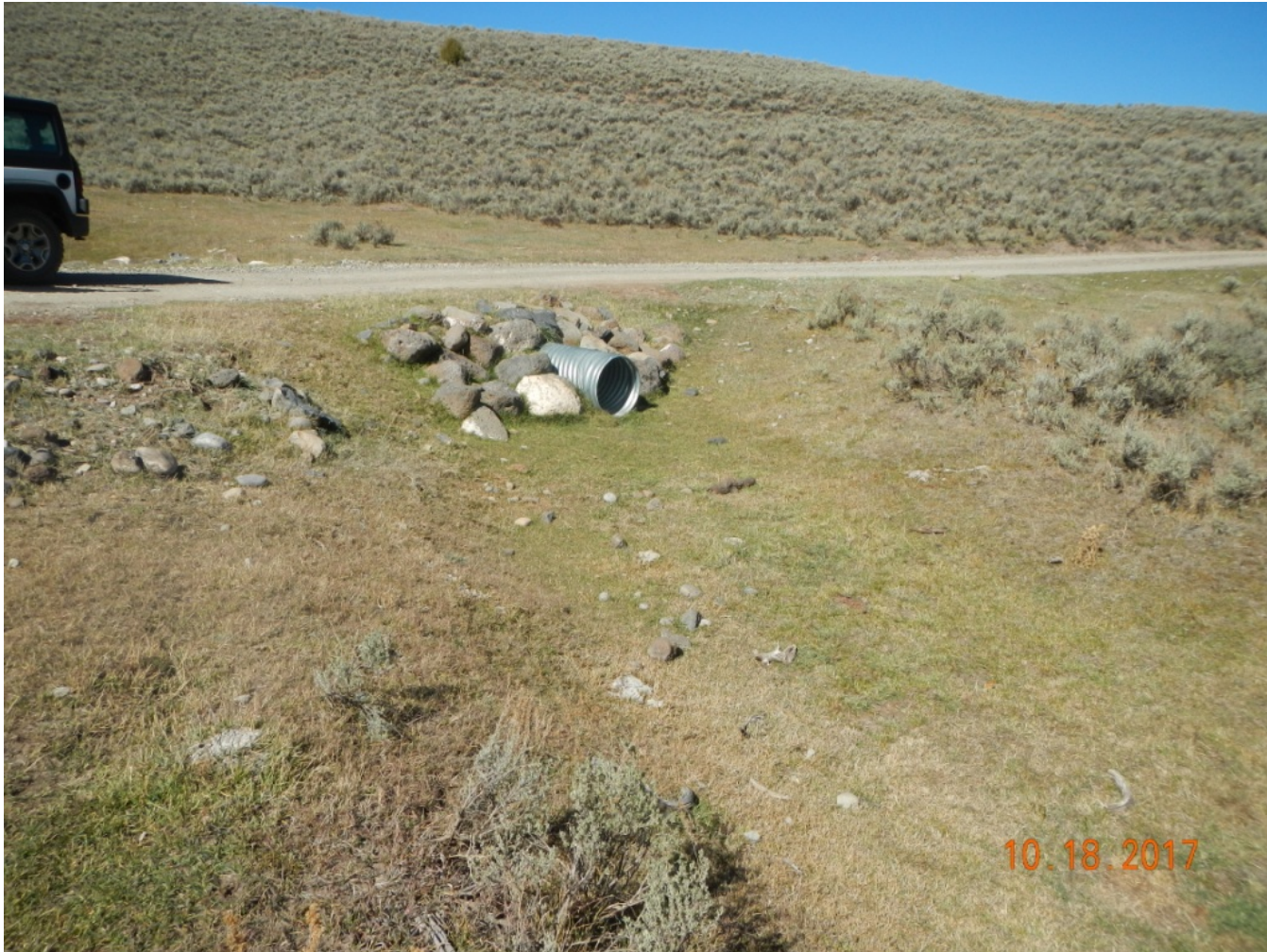
Photo 7. View of culvert along the access road that is in good condition.
