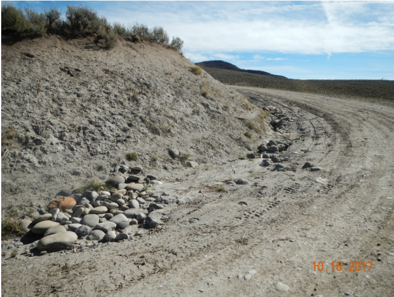
Photo 6. Another view of sediment filled rock check dams along the access road.
