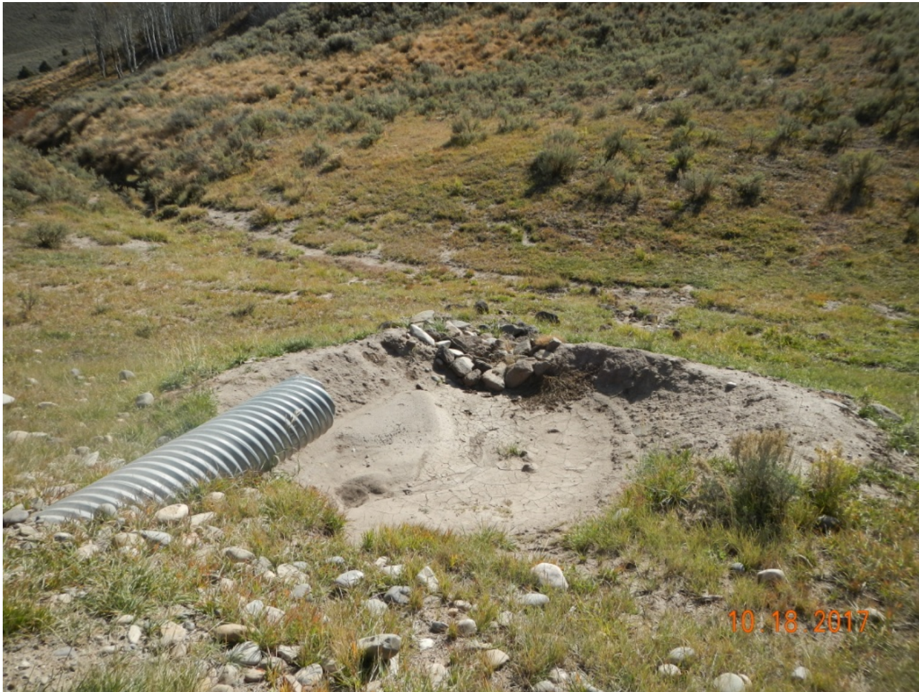
Photo 7. View of silt trap at culvert outlet along the access road.
