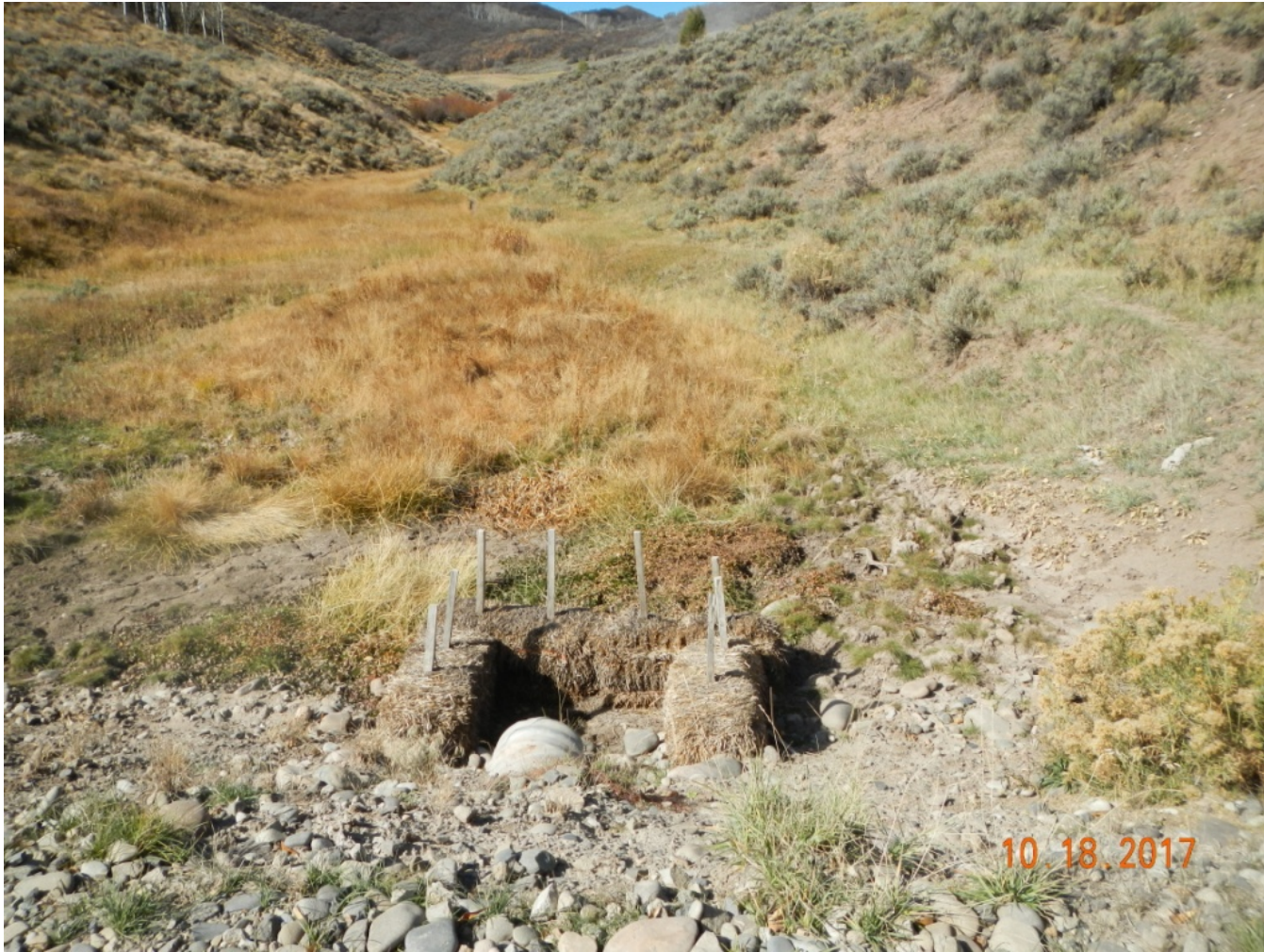
Photo 8. View of sediment controls at culvert at the lease road.
