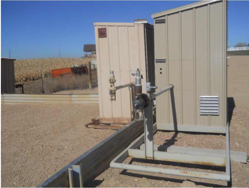
2-unused/disconnected gas meter runs east of separator
