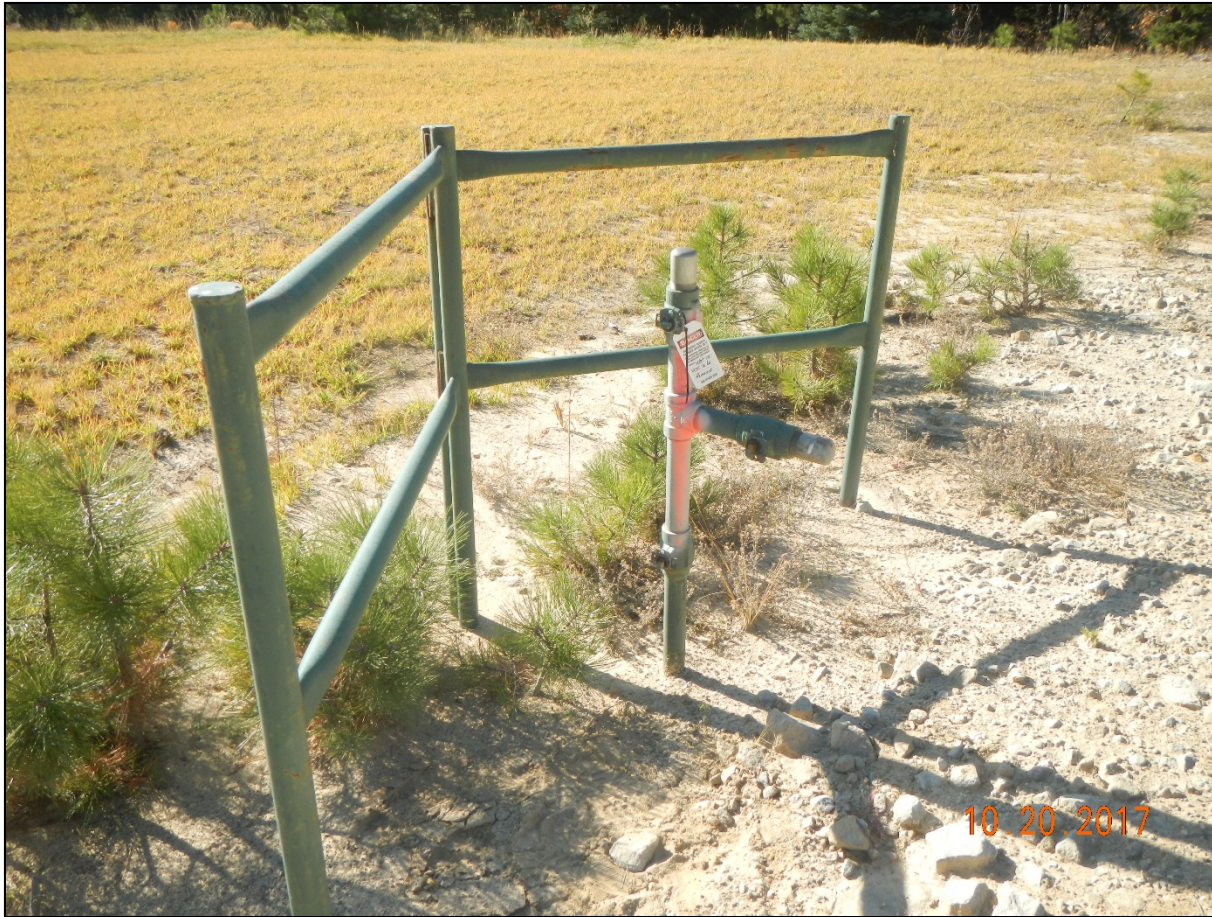
Photo 9. There is a pipe riser that remains at the east side of the location which appears to be marked for removal.
