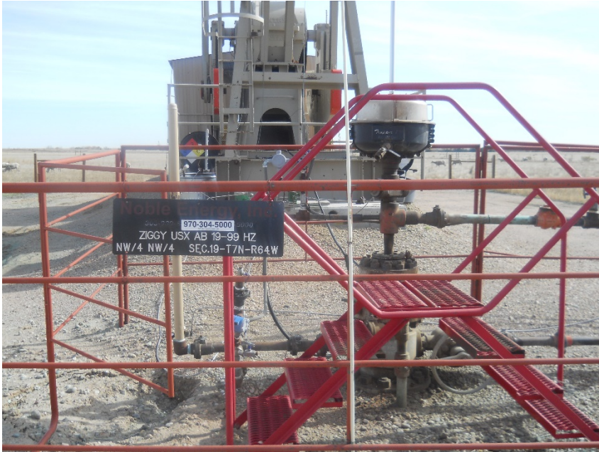
Wellhead looking east, stained soil around wellhead
