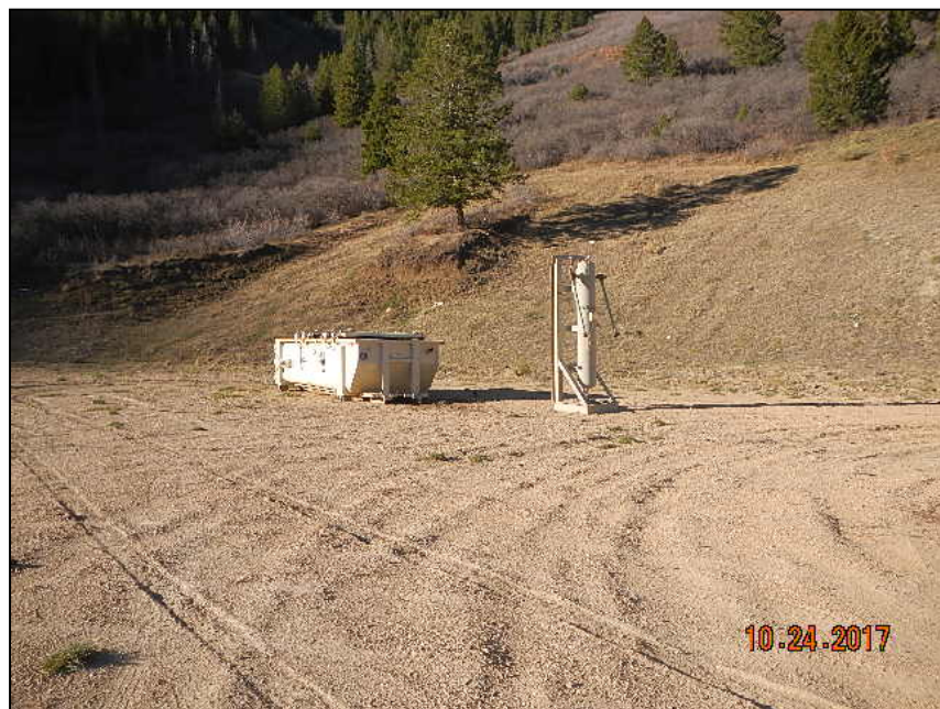
Photo 1. Tank and sand trap have been disconnected from well but not removed from site as stated in FIRR Doc#401438181 CA# 104930 and 104931
