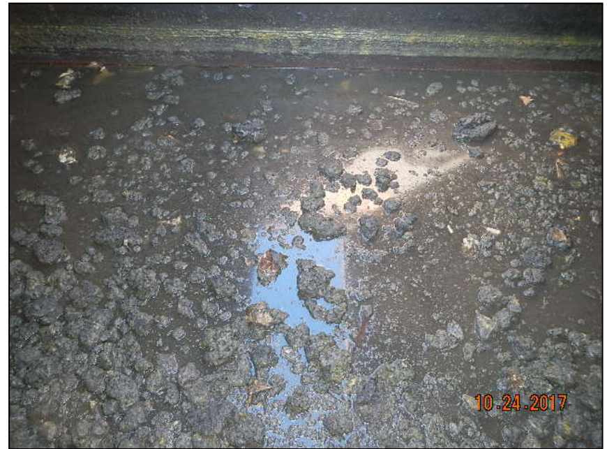
Photo 4. Tank contained sand AND produced water.
