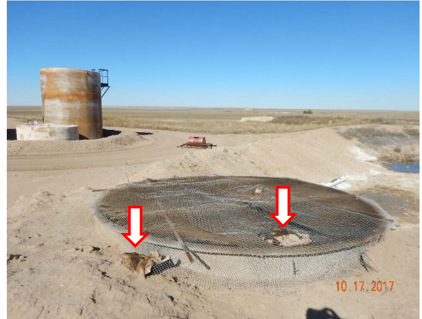
Photo #22 – Open-top skim tank at SE corner of production facility. Note oily rag and small pile of oily waste. Tank lacks NFPA placard and volume/content labels.
