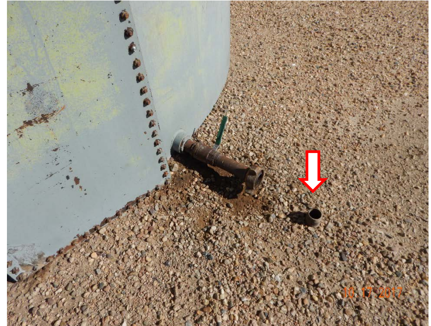
Photo #14 – Localized, oil-stained soil and 2" pipe riser beneath uncapped valve on west side of northern crude oil AST.
