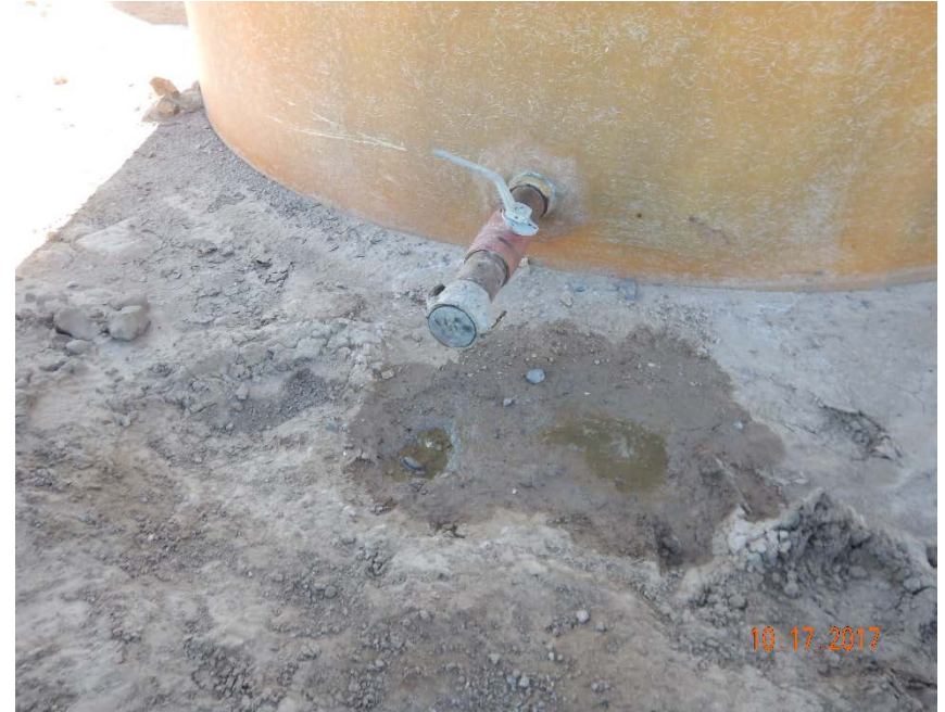
Photo #18 – Puddle of water at 300 bbl produced water AST loadout.
