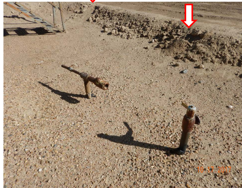
Photo #16 – 2" steel flowline risers SE of crude oil ASTs. Note that berms in background are eroded and damaged.
