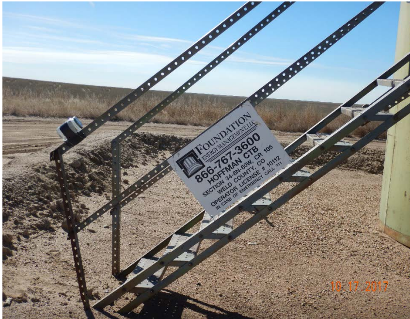
Photo #11 – Battery sign and eroded berms at SE corner of crude oil ASTs.
