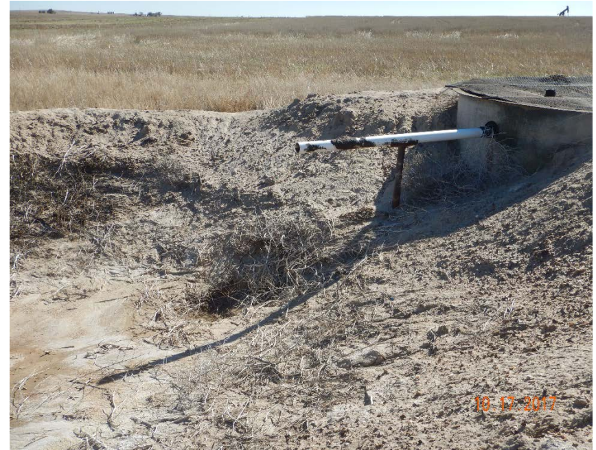
Photo #24 – Localized accumulations of oil-stained soil and weeds at SW corner of produced water pit #273442.
