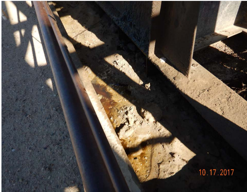
Photo #5 – Oil-stained soil and pooling fluid on west side of pump jack.
