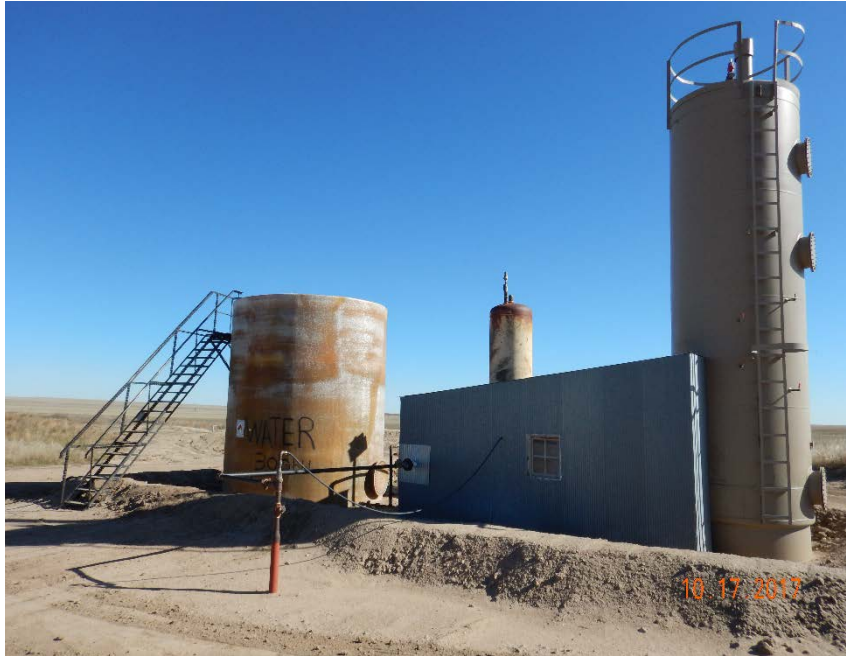
Photo #17 – Produced water AST and separator shed.
