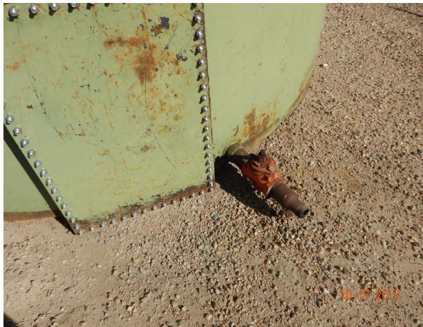
Photo #15 – Valve on west side of southern crude oil AST lacks bullplug.
