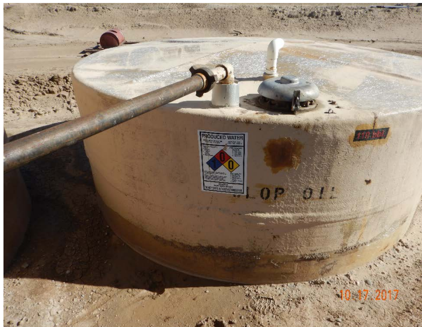
Photo #19 – 110 bbl produced water fiberglass PBV.
