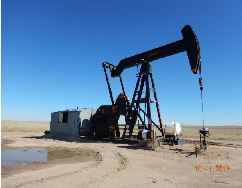
Photo #1 – View of wellhead and pump jack from the northwest. Note that precipitation is pooling on well pad.
