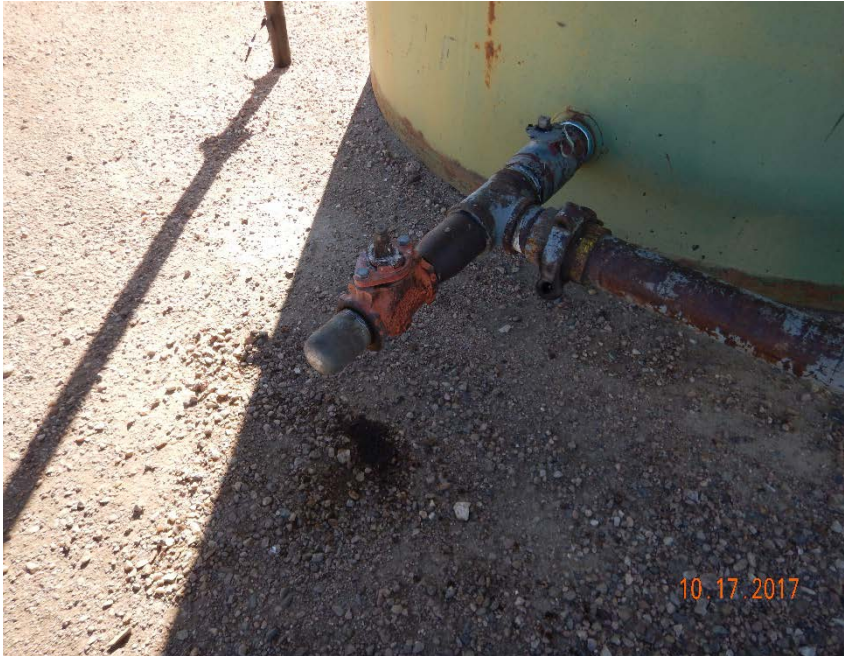
Photo #13 – Localized, oil-stained soil at crude oil AST loadout valve.
