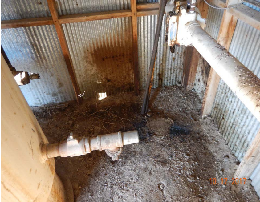
Photo #21 - Localized accumulations of oil-stained soil inside of separator shed (2).
