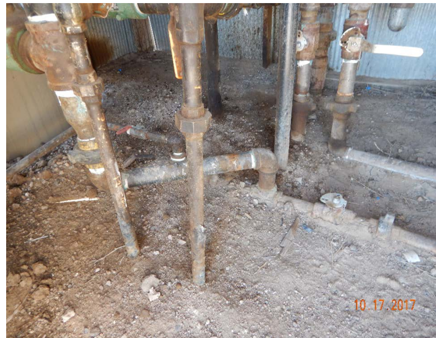
Photo #20 – Localized accumulations of oil-stained soil inside of separator shed (1).
