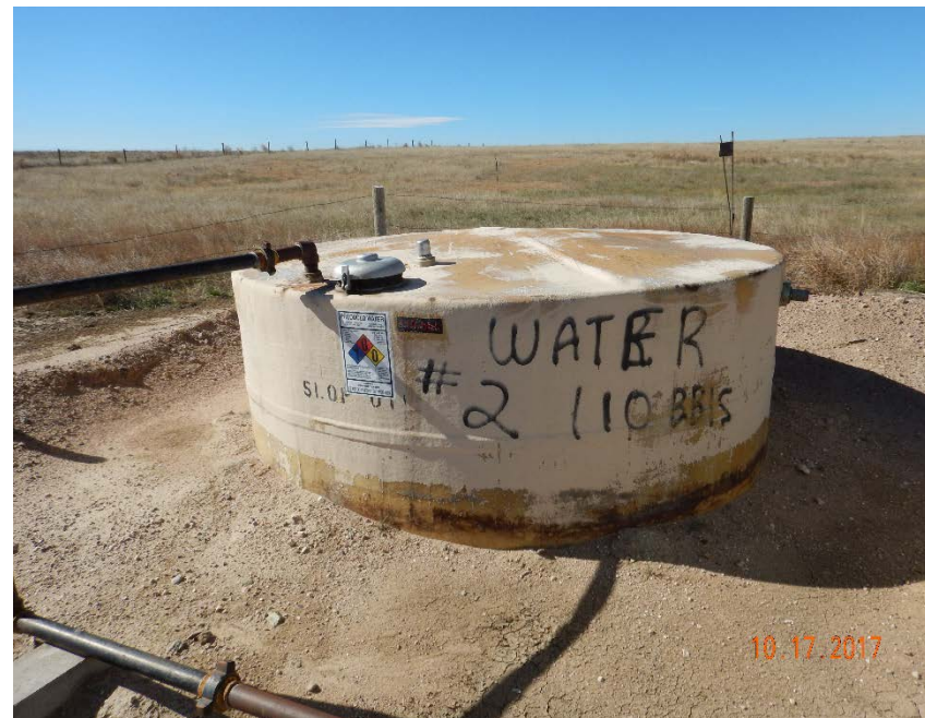
Photo #22 – 110 bbl fiberglass PBV SW of separator shed.
