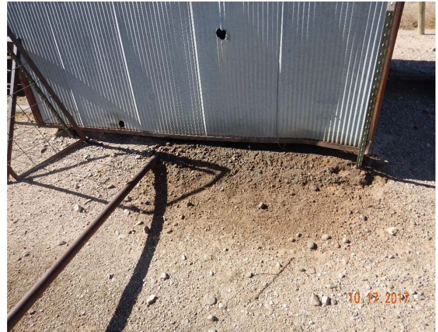
Photo #6 – Localized, oil-stained soil seeping from east side of shed.
