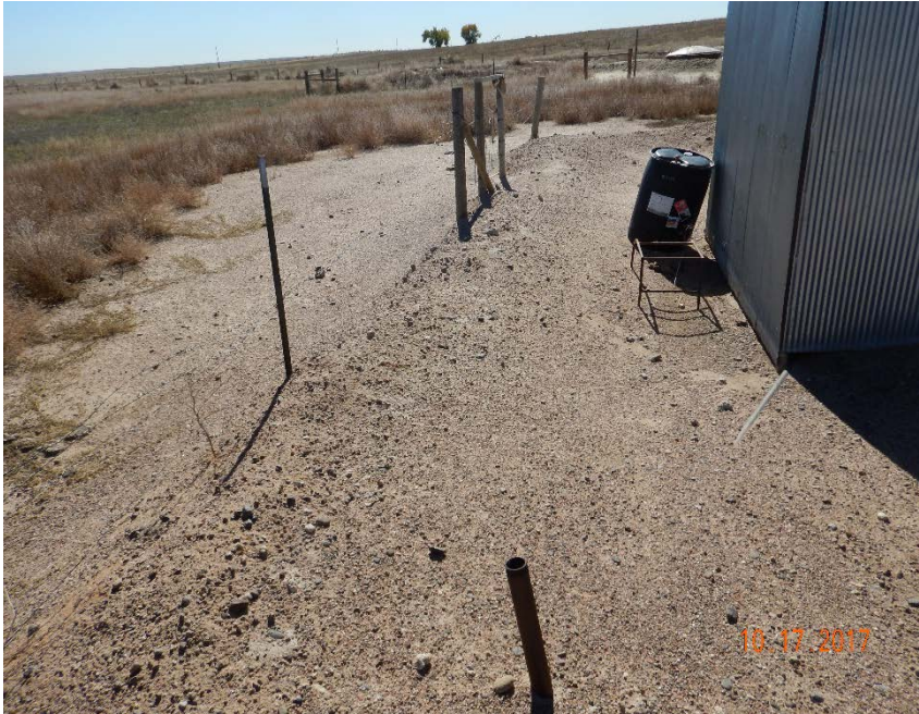
Photo #17 - 55-gallon drum lacking secondary containment and damaged barbed wire fence on east side of separator shed. Note uncapped 2" pipe riser in foreground.
