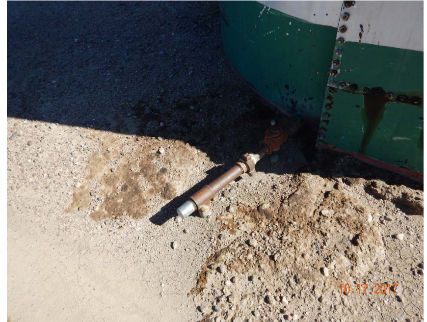
Photo #10 – Historical accumulation of oily waste beneath valve on west side of crude oil AST.
