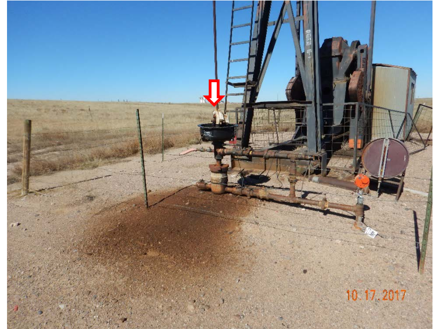
Photo #2 – Oil-stained soil at wellhead and day tank lacking secondary containment at SE corner of pump jack. Note oily rag attached to polished rod/wellhead and damaged panel fence at shed.
