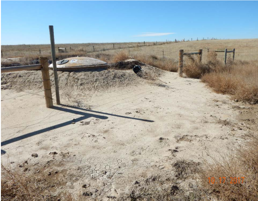
Photo #25 – Off-site sediment transport from pit berm onto area north of pit fence.
