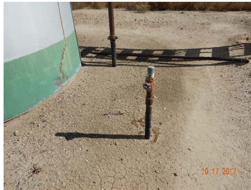
Photo #12 – Bullplugged 2" riser south of crude oil AST.
