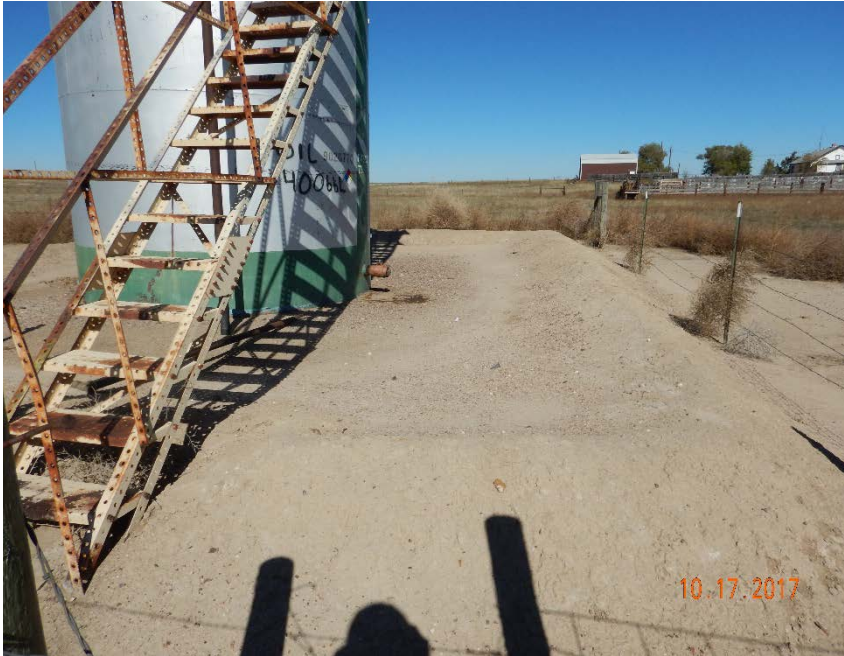
Photo #9 – Localized accumulation of oily waste beneath valve on east side of 400 bbl crude oil AST. Note proximity of production facility to inhabited buildings to NE.
