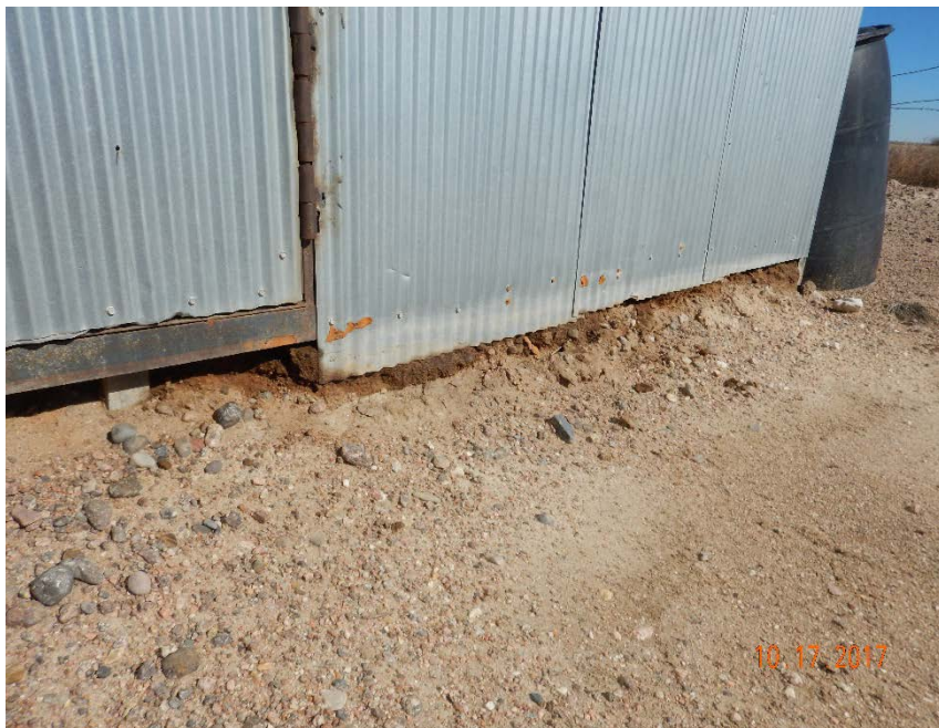
Photo #19 – Historical accumulation of oily waste beneath SE corner of separator shed.
