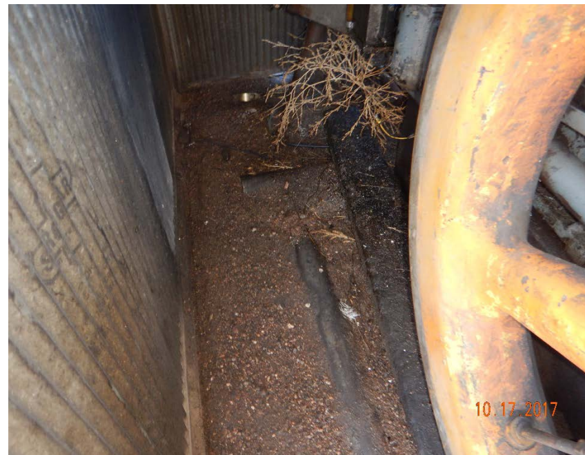
Photo #8 - Oil-saturated soil beneath prime mover (2).
