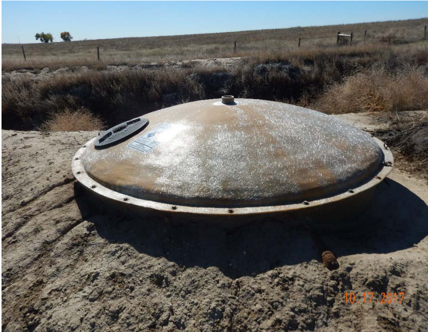
Photo #27 – Fiberglass skim tank lacks earthen berms on west, north, and east sides as well as volume label.
