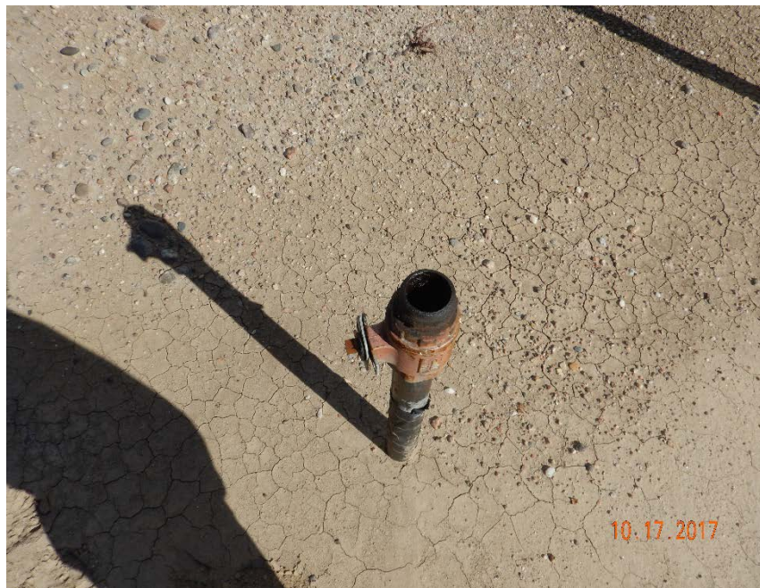
Photo #11 – Uncapped 2" flowline riser SW of crude oil AST.
