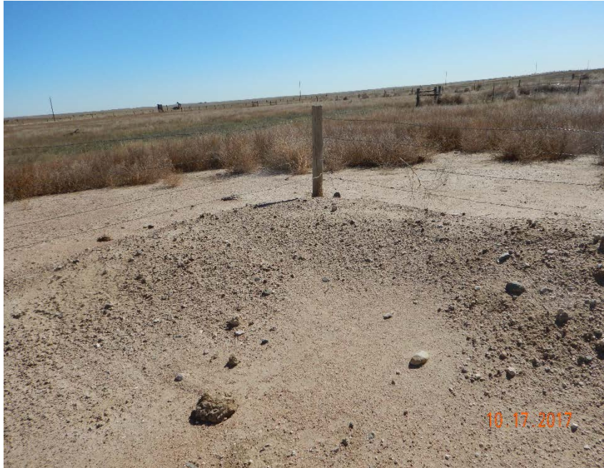
Photo #23 – Earthen berm for fiberglass produced water PBV is shallow at SE corner.
