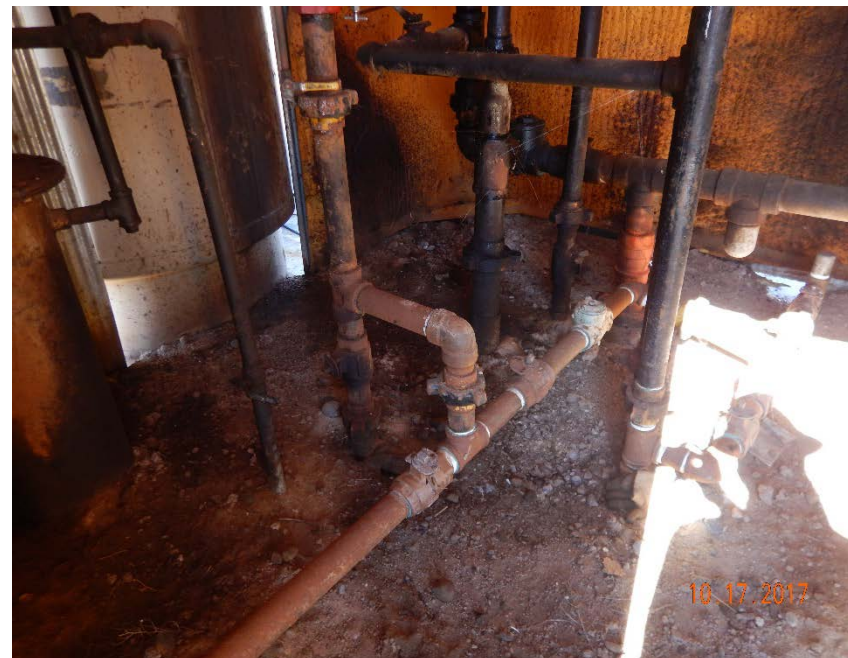
Photo #20 – Oil-stained soil and historical accumulations of oily waste inside of separator shed (1).
