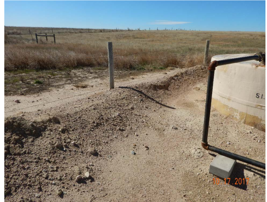
Photo #24 – Earthen berm for fiberglass produced water PBV is shallow south of tank.
