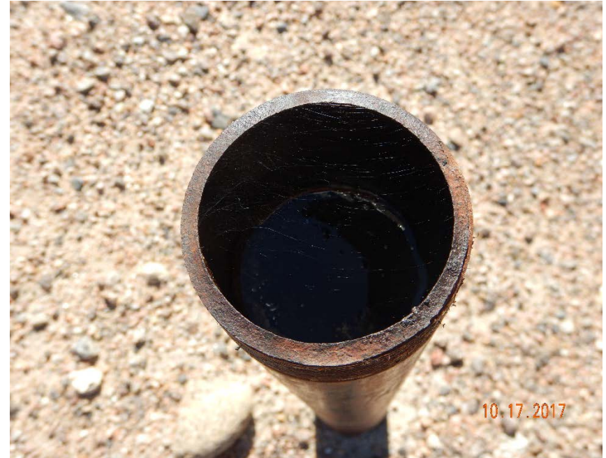
Photo #18 – Uncapped 2" pipe riser NE of separator shed contained crude oil.
