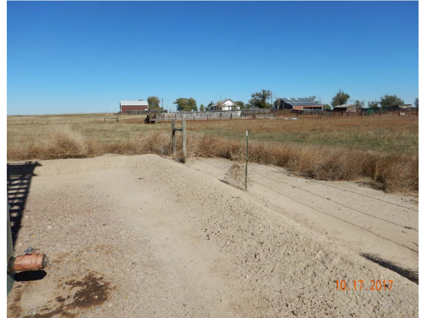
Photo #14 - Shallow, eroded earthen berm NE of crude oil AST and proximity to occupied buildings NE of production facility.
