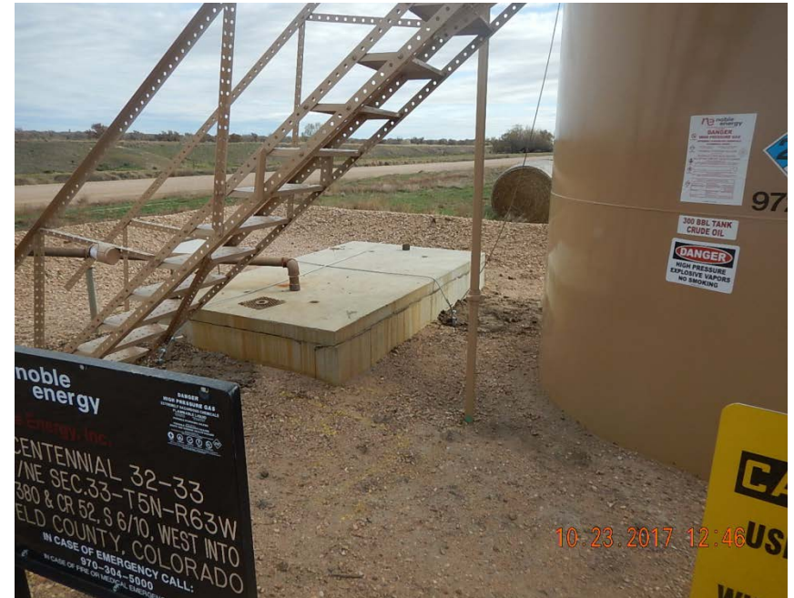
Photo 4: Concrete vault anchored. Berm is earthen in floodplain.
