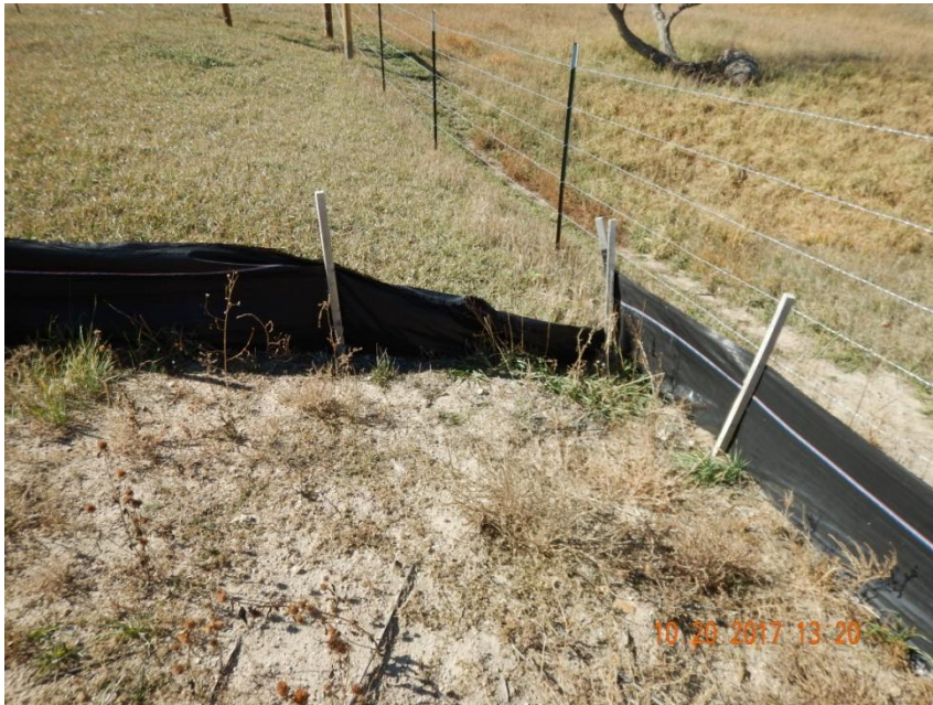
Photo 5. Photo taken from the southeastern location, facing South. BMP maintenance needed along a section of the silt fence. Photo illustrates no further work has been conducted as of October 20, 2017.
