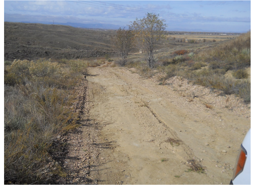
Access road from wellhead to battery looking northwest. Still washing out 10-23-2017
