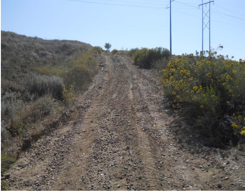
Access road to wellhead from battery looking southeast. Road is washing out on both sides 9-12-2017
