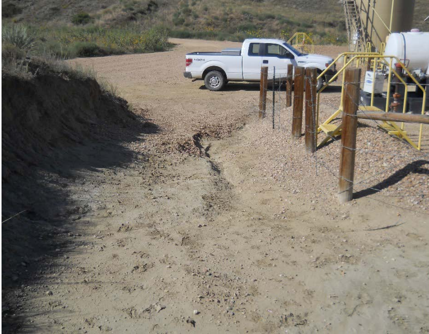
Location washing out south side of separator 9-12-2017
