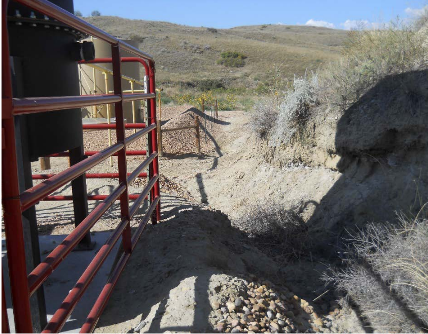
Location washing out north side of location, discharging northwest of tank battery with sediment carrying off into field 9-12-2017
