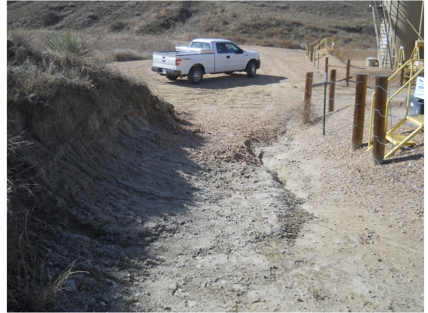
Location washing out south side of separator 10-23-2017
