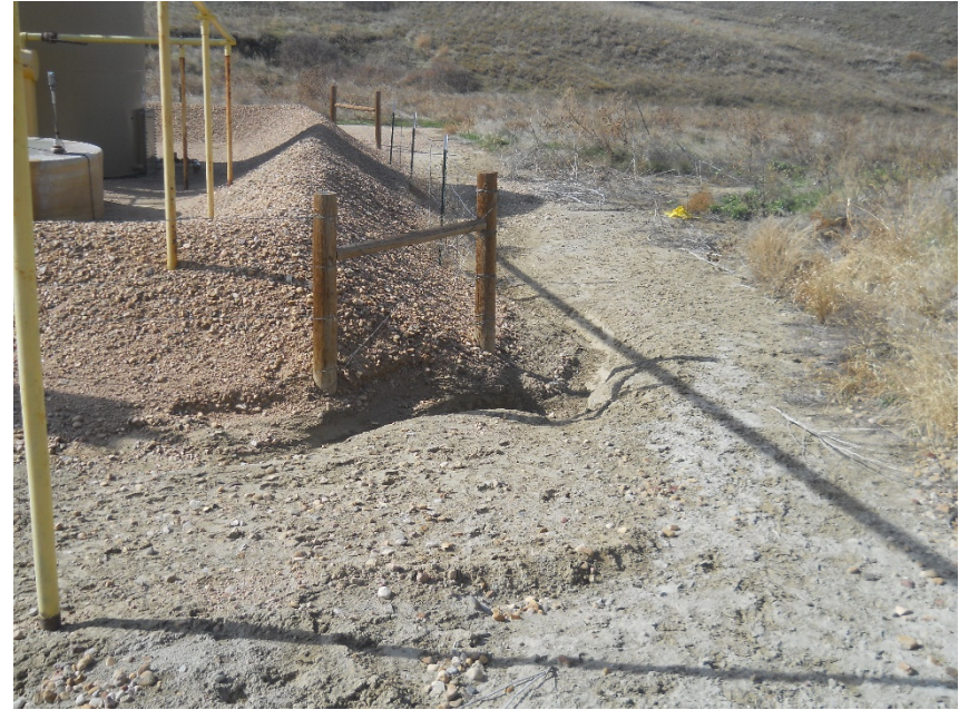
Northeast edge of tank battery is washing out 10-23-2017
