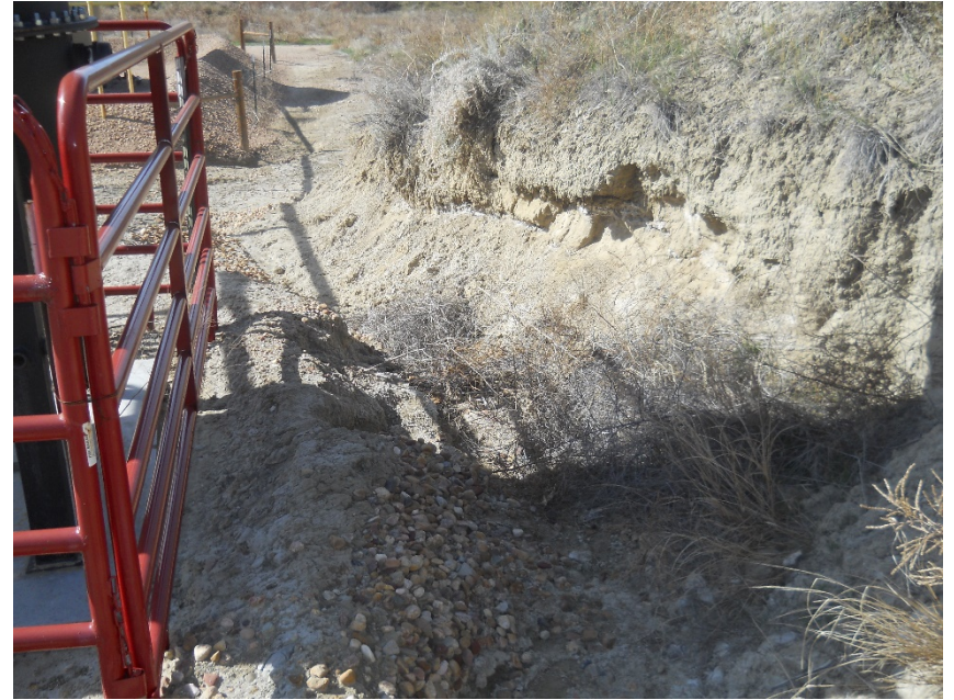
Location washing out north side of location, discharging northwest of tank battery with sediment carrying off into field 10-23-2017
