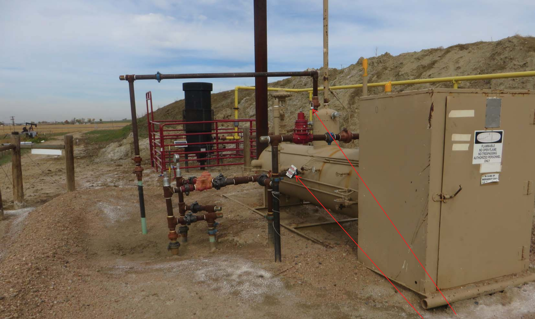
battery 452625 separator and combustion device with inlet and outlet valves to separator closed and locked out
