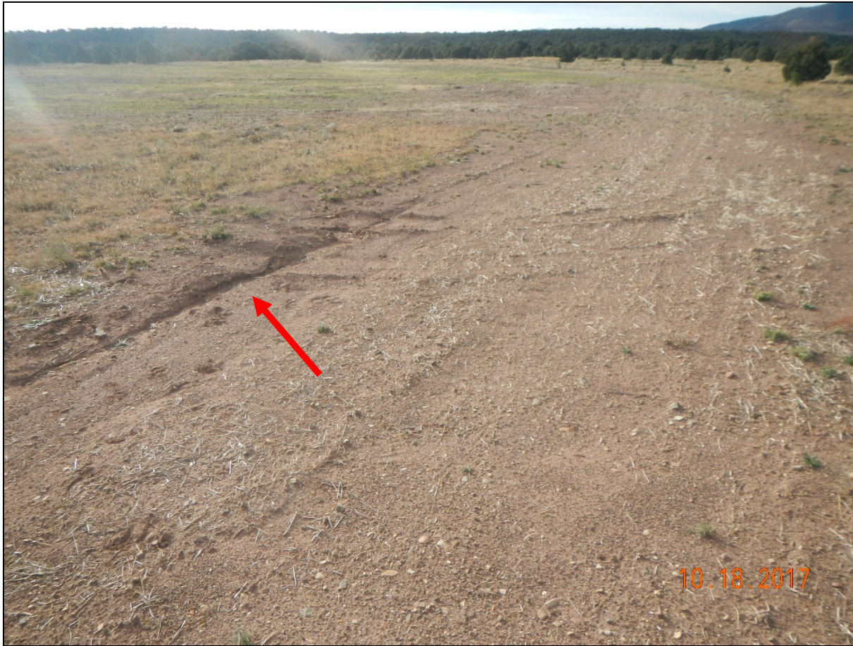
Photo 8. Facing south where the unpermitted disturbance occurred. The area where the access road was built does not have vegetation establishment. The soils appear to be compacted. The red arrow points toward an area of stormwater erosion rill.
