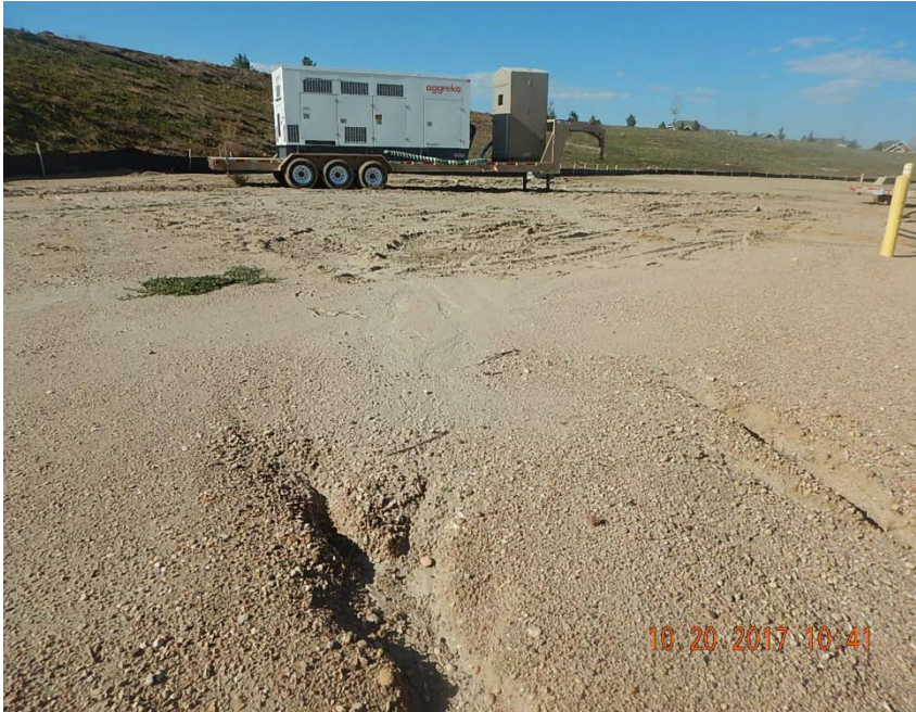
Photo 7: Stormwater erosion on W side of battery, looking W
