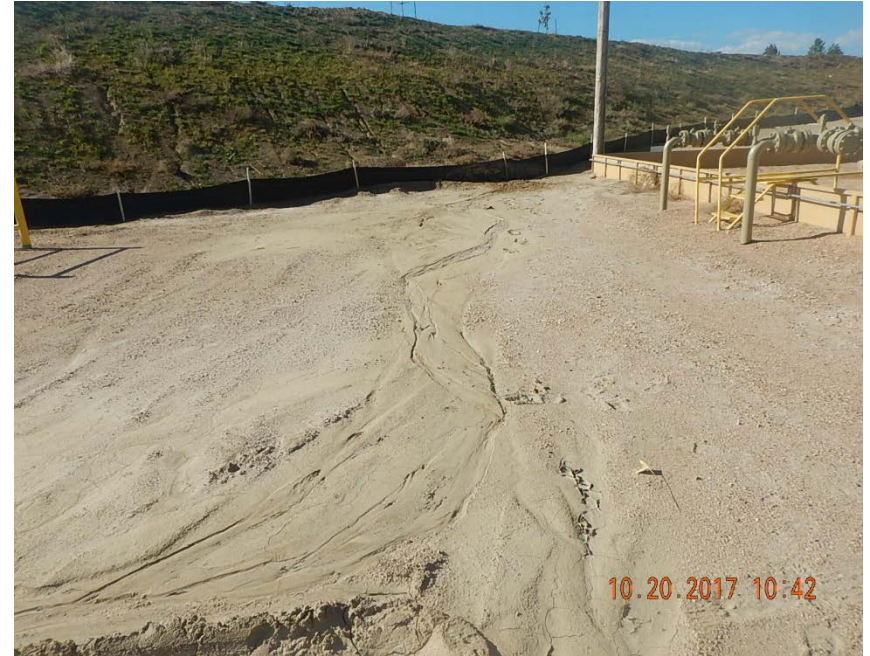
Photo 8: Stormwater erosion on S side of location, looking W
