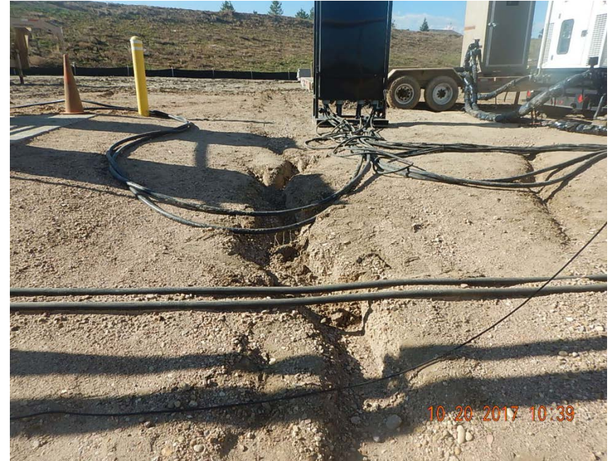
Photo 6: Stormwater erosion at SW corner of location, looking W
