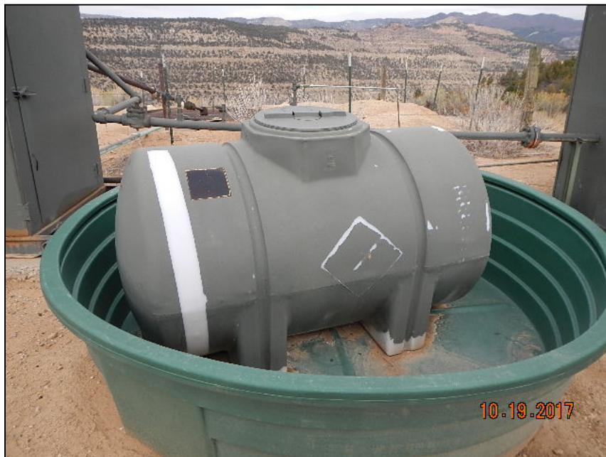
Photo 1. Signs on tank not legible.
