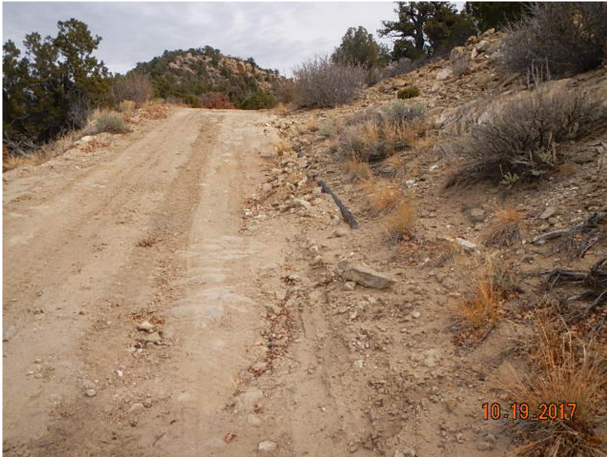
Photo 1. Access road to location has multiple areas of erosion and sediment migration down gradient of road surface and exposed pipeline.
