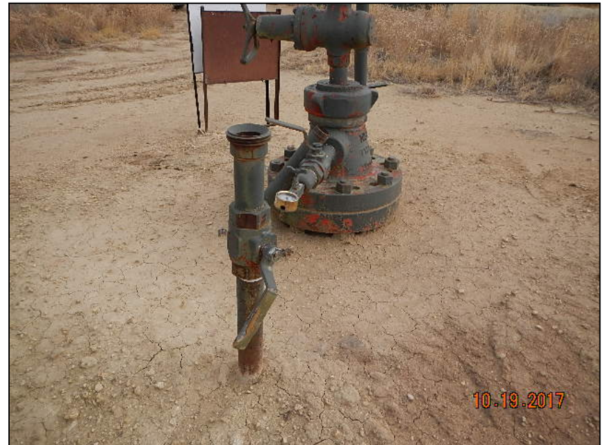
Photo 2. Unmarked riser at wellhead.
