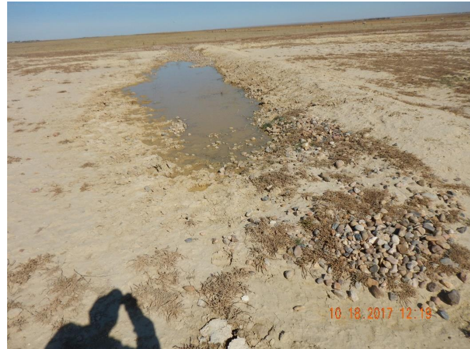
Photo 25: Photo taken from the south end of the disturbance, facing north. Photo shows what appears to be a berm used to pond stormwater installed by the operator. Rock aggregate at base of BMP has filled with sediment.
