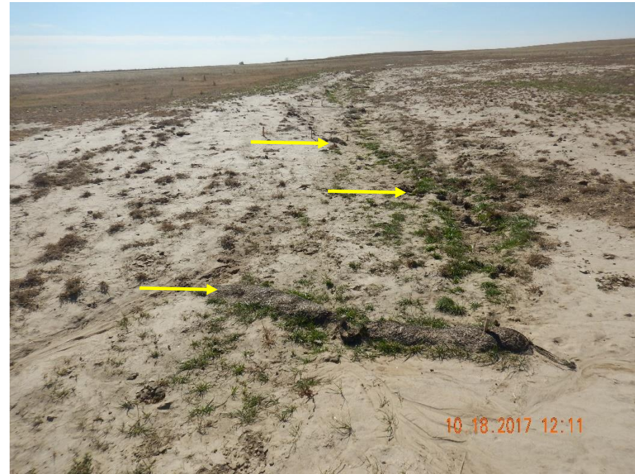
Photo 15: Photo taken from the south end of the berm in photos 11-14, facing south. Photo shows a drainage where operator had installed straw wattles. Wattles observed here were in disrepair and no longer in proper functioning condition. Stormwater BMPs have not been maintained.
