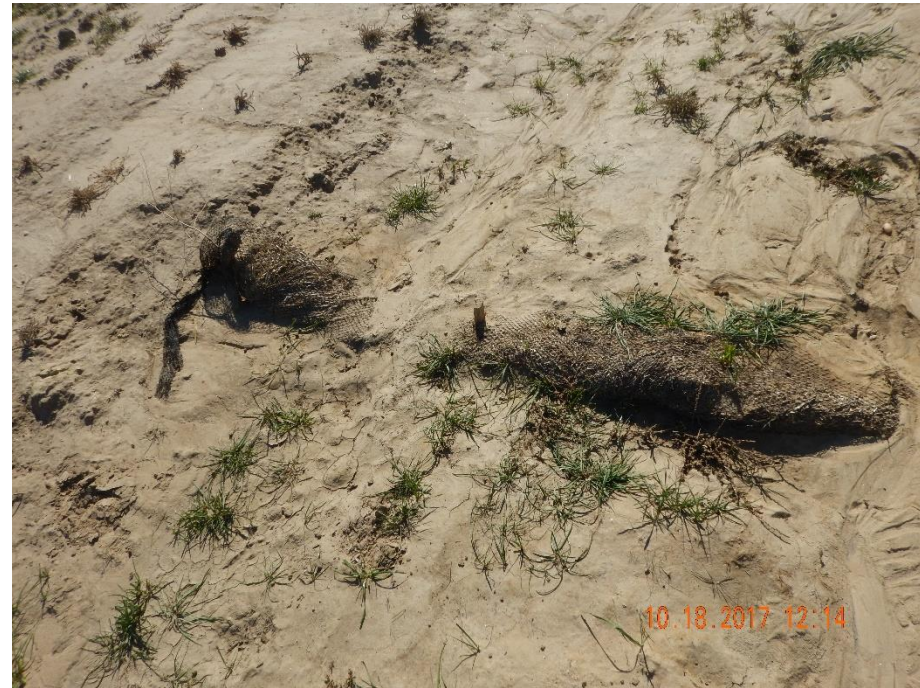
Photo 17: Continued from photo 16. Photo show straw wattle in disrepair.
