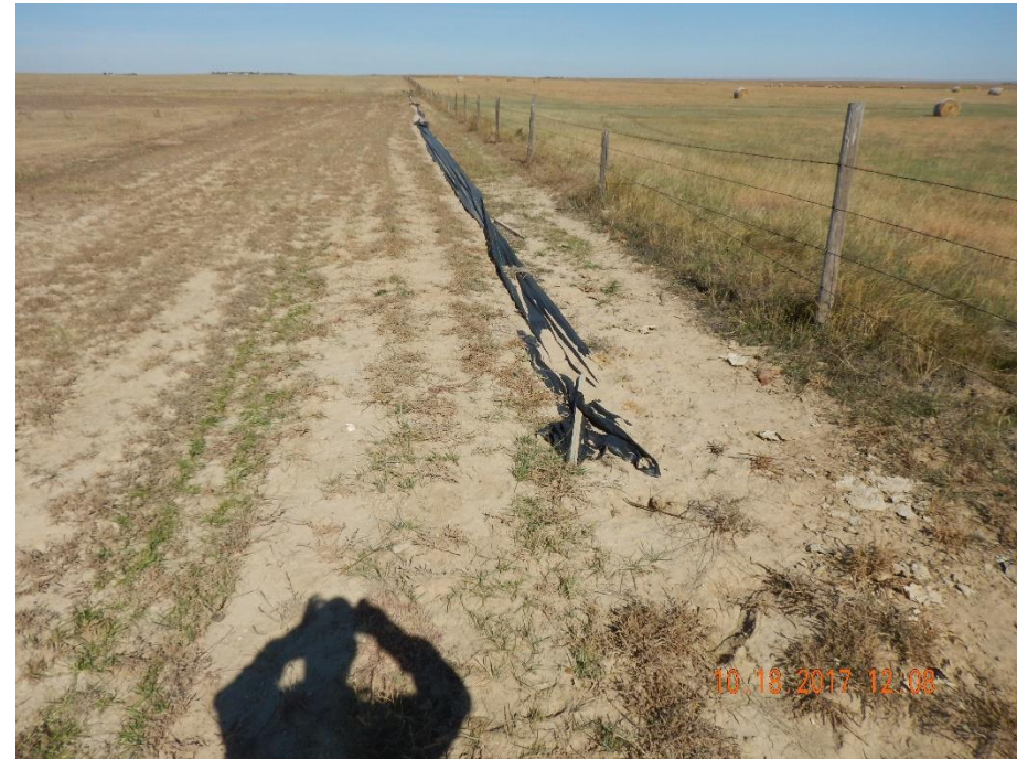
Photo 7: Photo taken from the east end of the disturbance, facing north. Photo shows silt fence BMP that is in disrepair and no longer in proper functioning condition.
