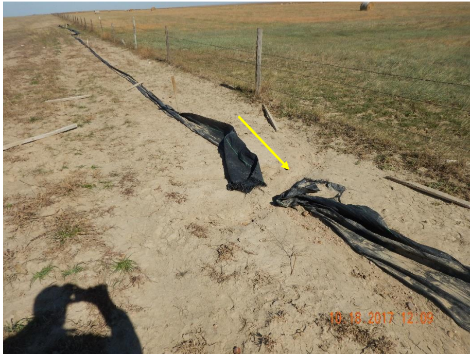
Photo 8: Photo taken from the east end of the disturbance, facing north. Photo shows silt fence BMP that is in disrepair and no longer in proper functioning condition. Photo also shows gulley erosion beginning to reform and lead onto adjacent lands.
