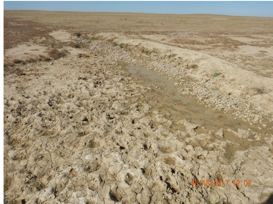
Photo 5: Photo taken from the east end of the location, facing west. Photo shows what appears to be a berm, with rock aggregate at the base to trap sediment. Aggregate appears to have filled with sediment in areas. Portions of the BMP on the east end (see photo 6) have eroded out.
