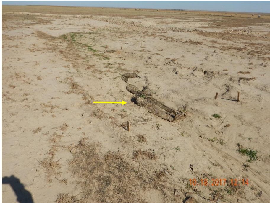
Photo 16: Additional photos continued from photo 15 showing straw wattle BMPs in disrepair. These wattles are now debris and needs to be repaired or removed and properly disposed.
