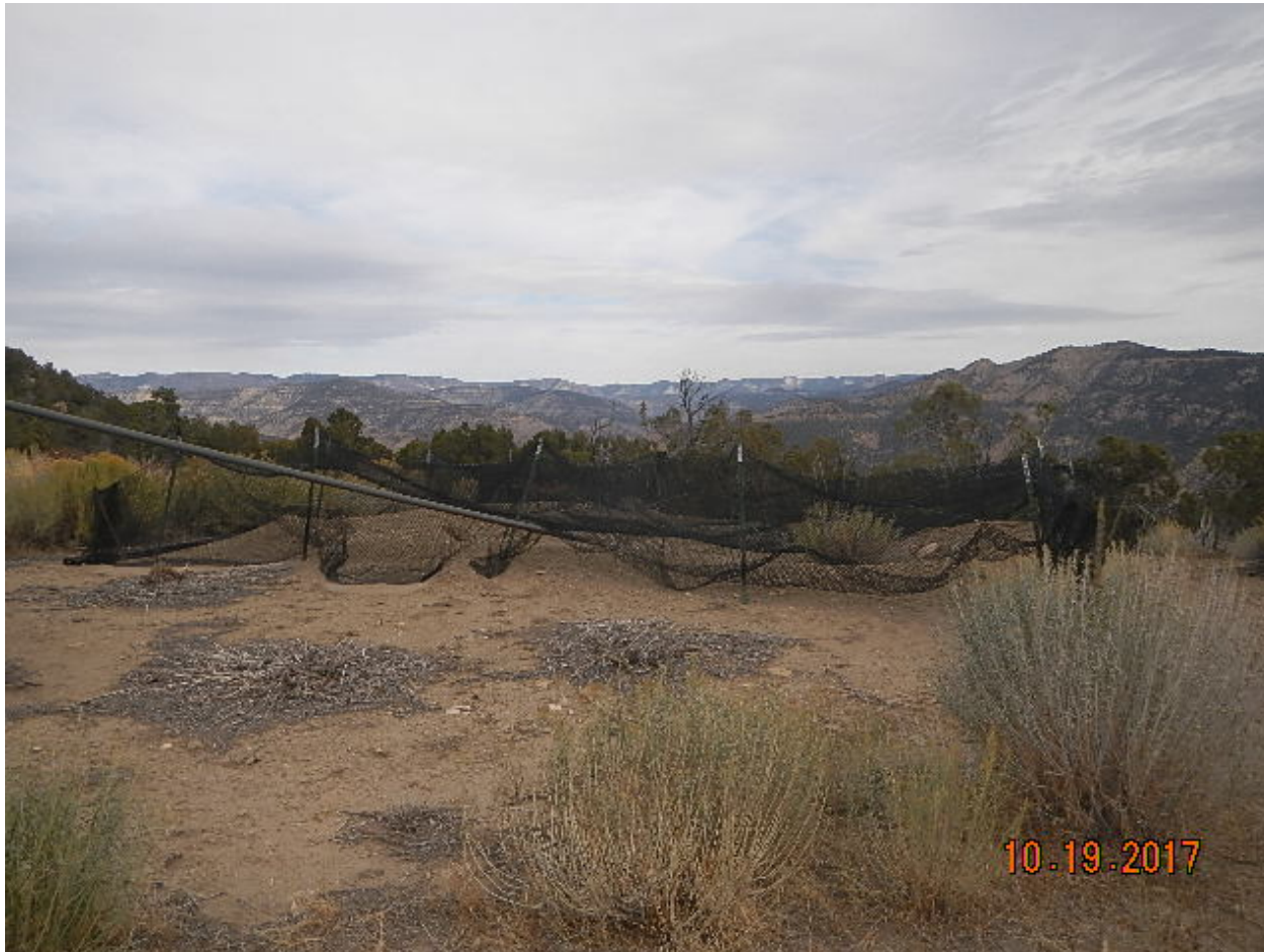
Photo 1. Netting on pit has not been maintained.
