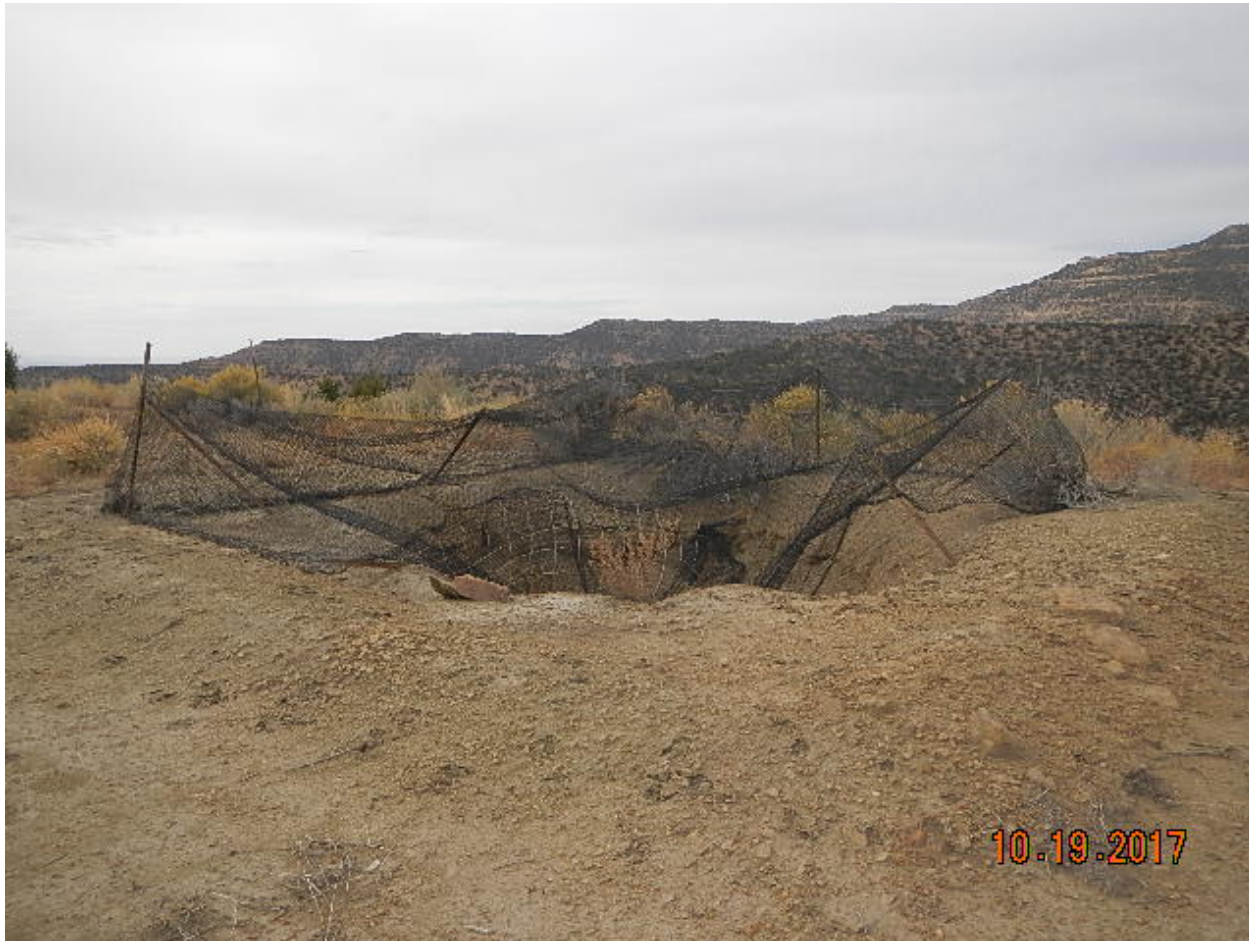
Photo 1. Fence and netting has not been maintained for pit.
