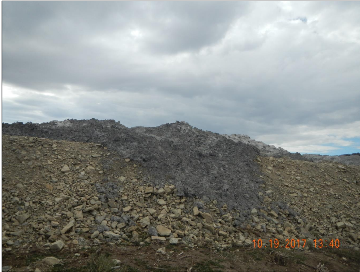
Cuttings over perimeter berm.
