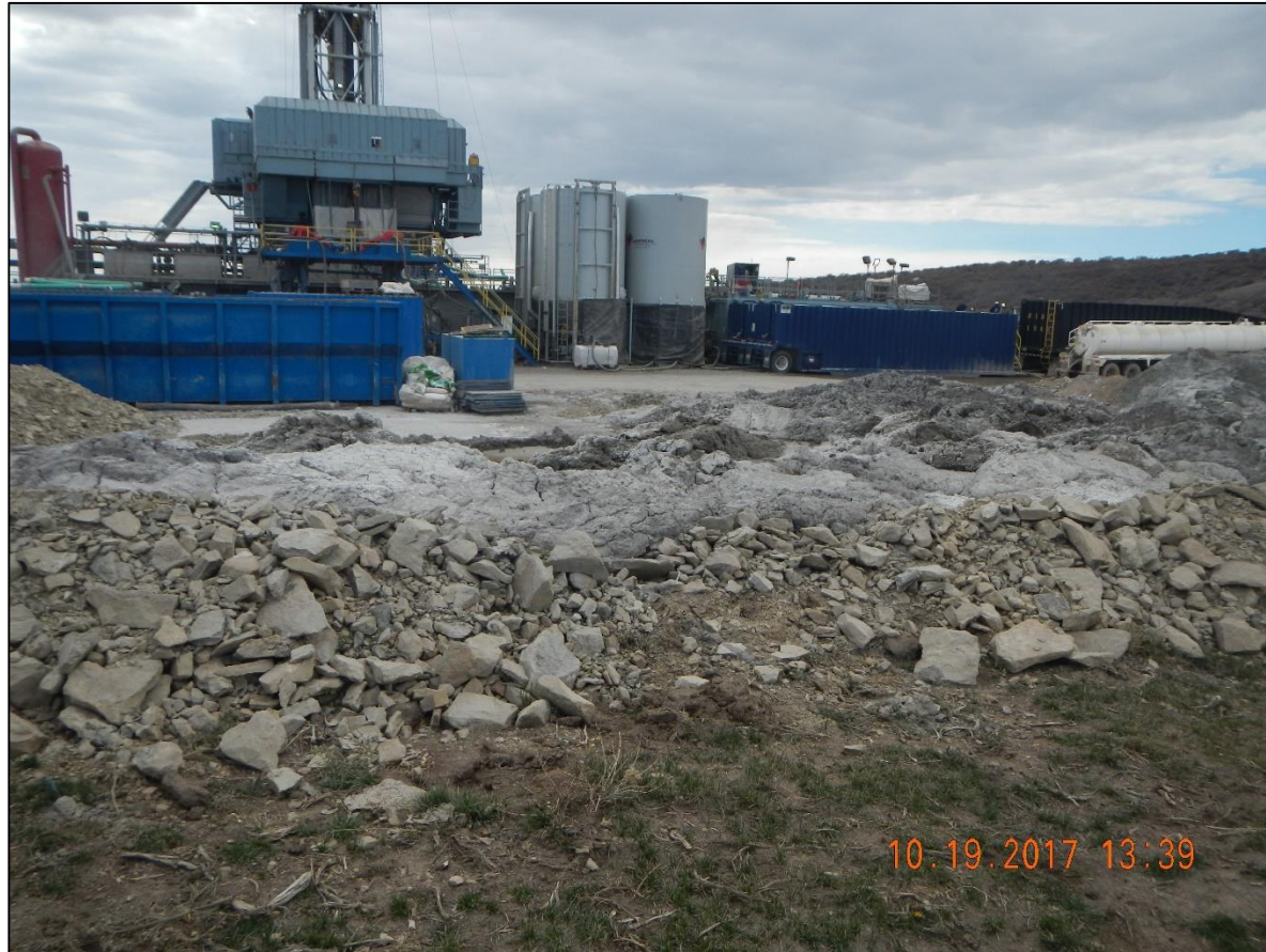
Cuttings over perimeter berm.
