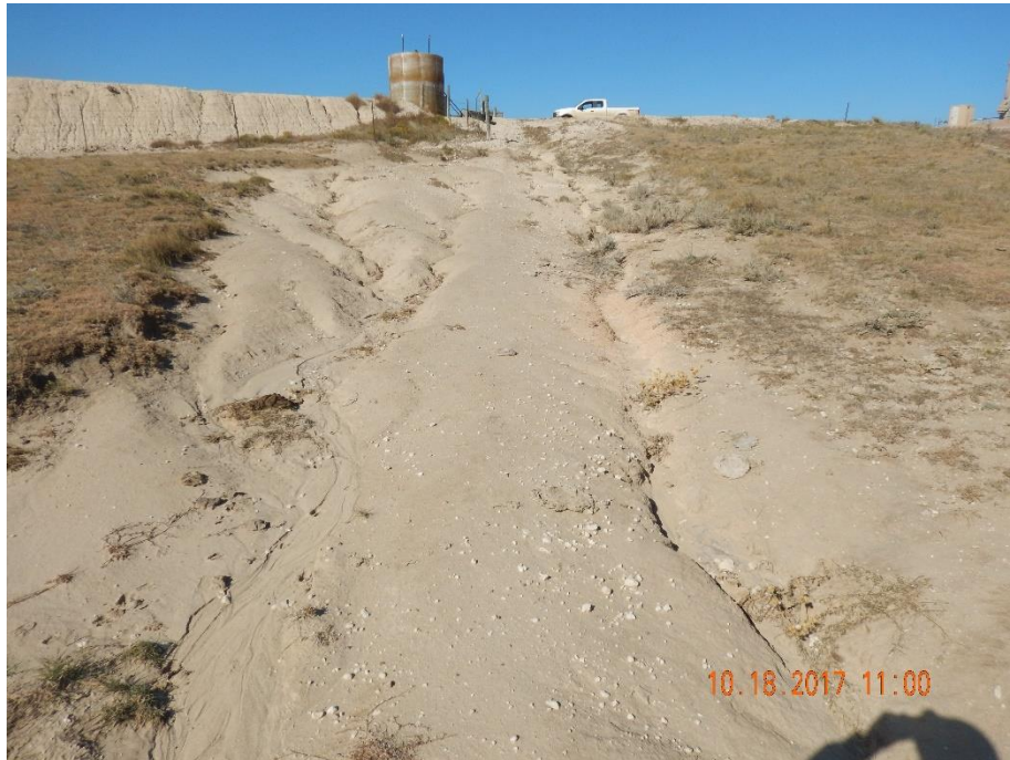
Photo 7: Photo taken from the northeast end of the pit, facing west. Photo shows no BMPs have been installed.
