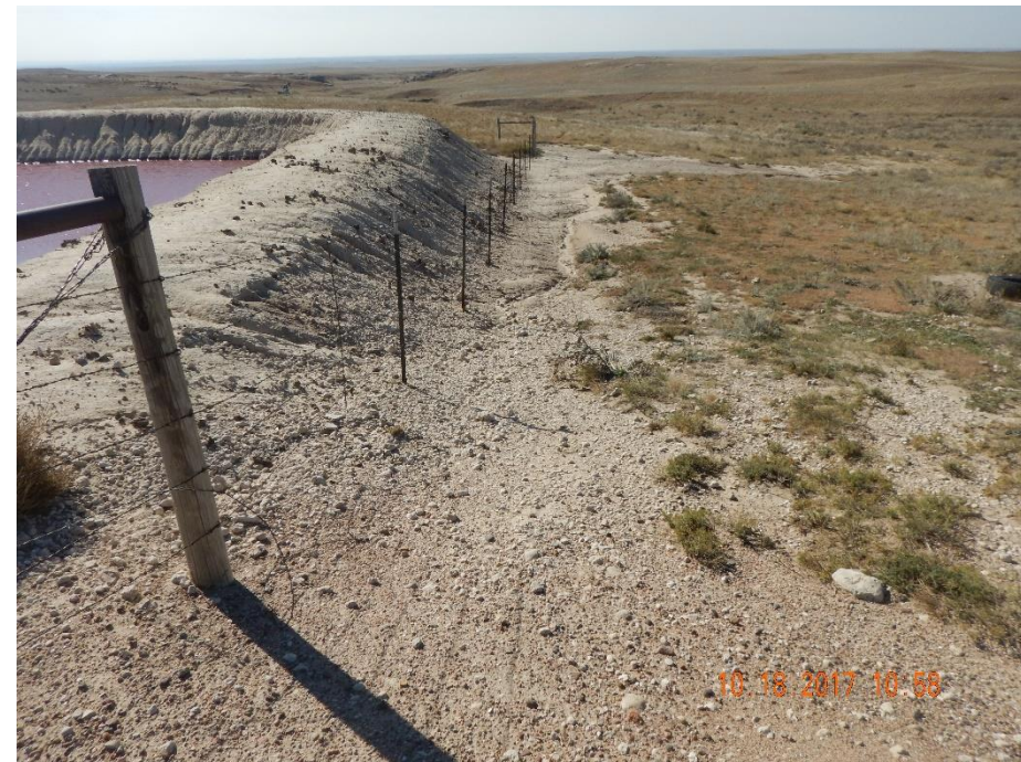
Photo 2: Photo taken from the northwest end of the pit. Photo shows erosion degradation. Previous inspection required operator to implement temporary stabilization controls. Photo shows no BMPs have been installed.
