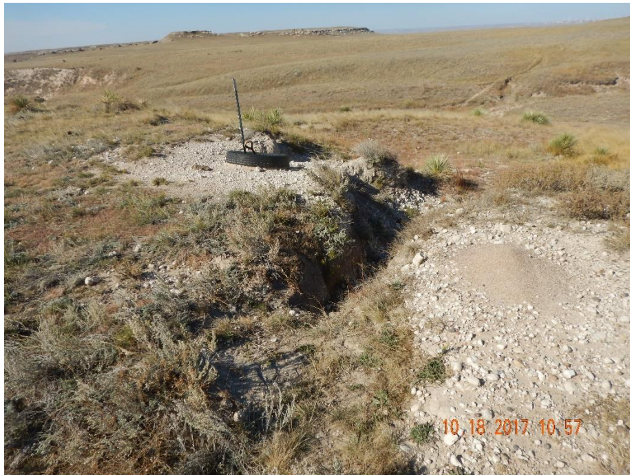
Photo 1: Photo taken from the west end of the location. Photo shows erosion degradation. Previous inspection required operator to implement temporary stabilization controls. Photo shows no BMPs have been installed.
