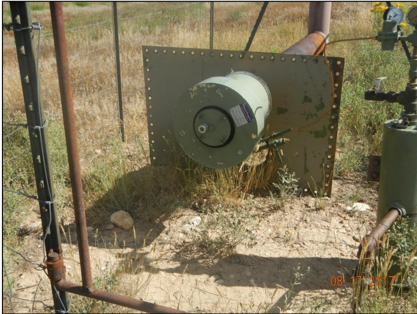
Combustible material around fired equipment 8.17.17 inspection photo
